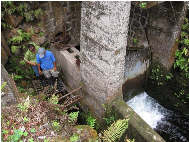
Figure. 2. Control gate at Waihe'e Ditch Intake on Waihe'e River. August 9, 2010.
