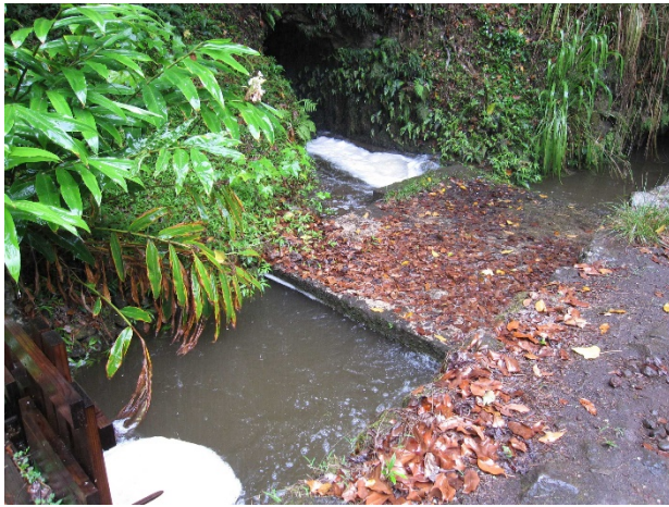
Figure 4. Water from Waihe'e Ditch Drop Ditch entering Spreckels Ditch on Waihe'e River. July 13, 2009.
