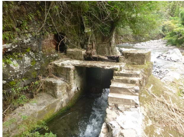
Figure 3. Spreckels Ditch Intake on Waihe'e River. March 5, 2018.
