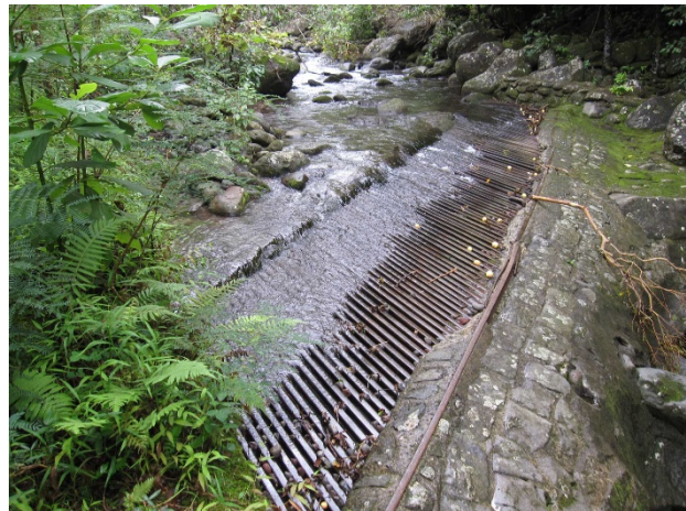
Figure 7. Waihe'e Ditch North Intake on Waihe'e River. November 1, 2011.
