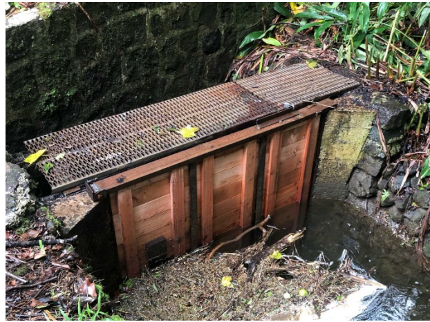
Figure 5. Control gate on Spreckels Ditch allows for water to be returned to Waihe'e River. January 10, 2020.
