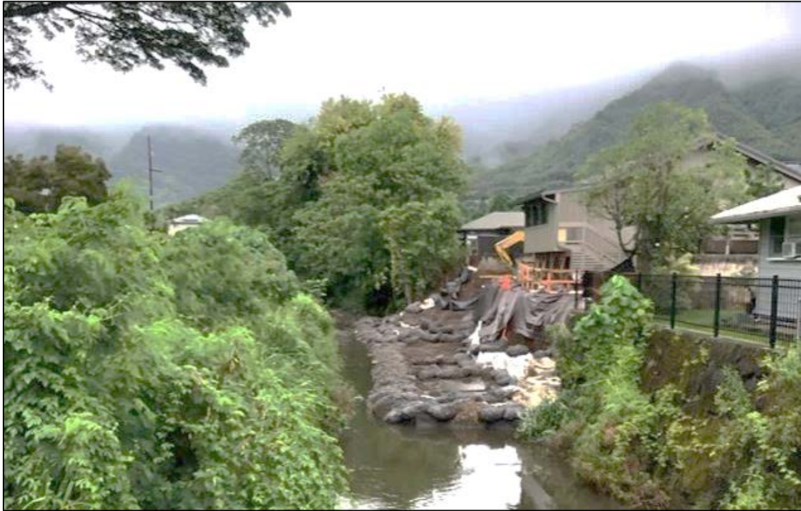
Site photo 1: Looking upstream taken from Kahaloa Bridge (staff, May 2019).
