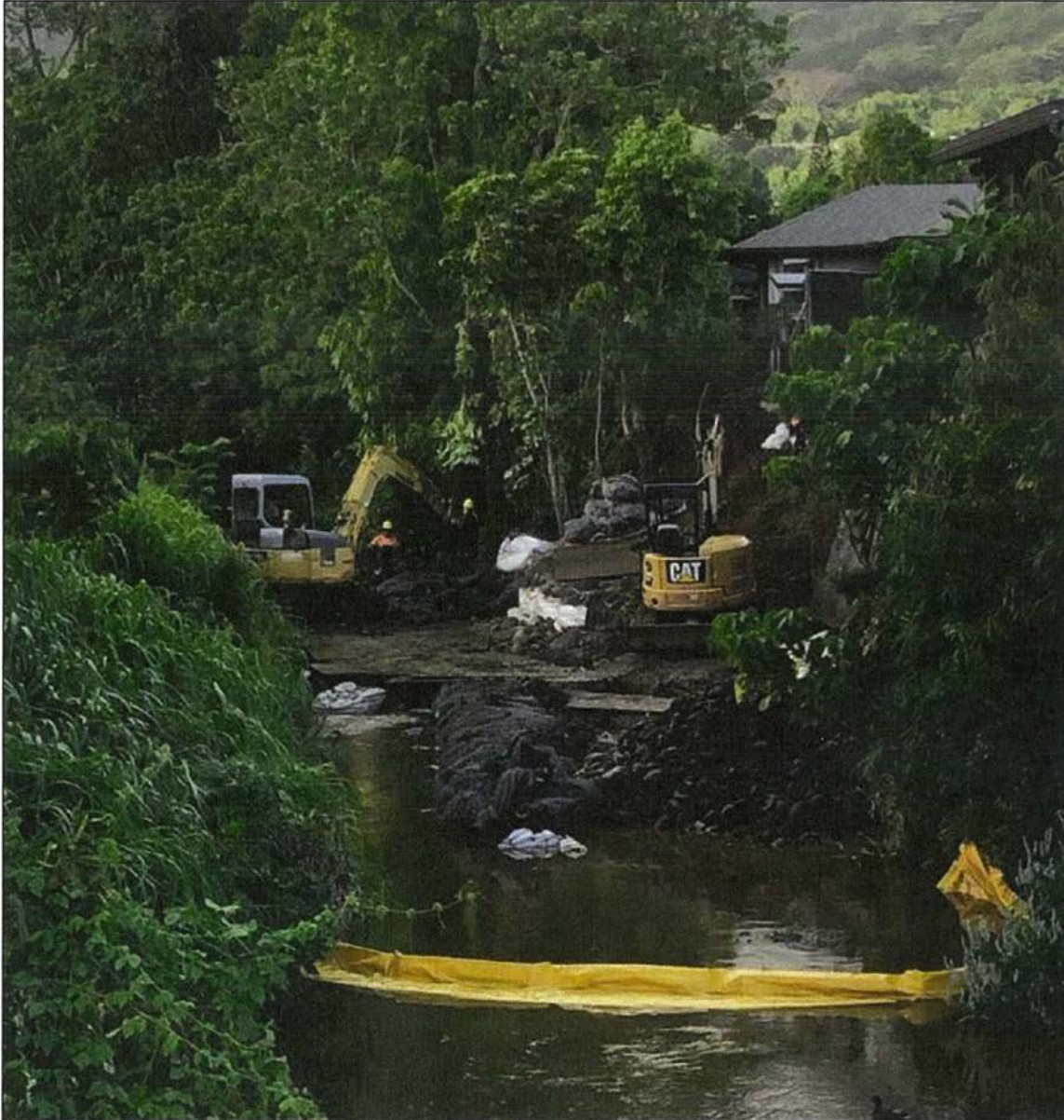
Exhibit 1: Site Photo of 3148C East Manoa Road, Manoa Stream, Manoa, Hawaii.
