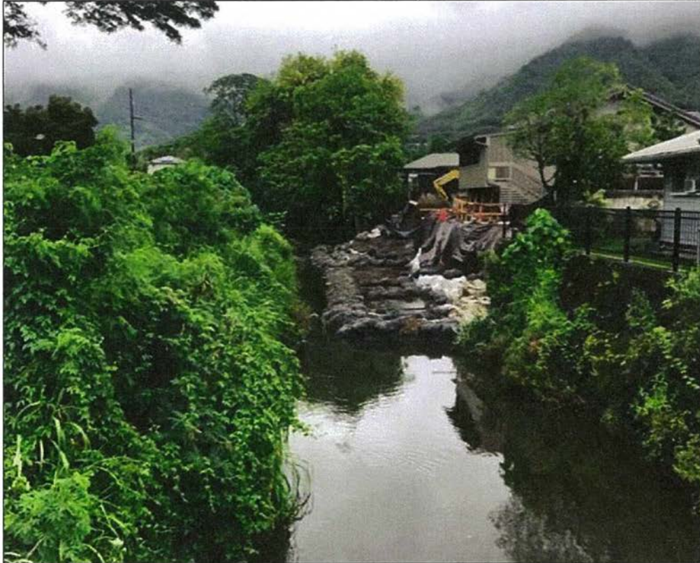
Exhibit 1: Site Photo of 3148 C East Mānoa Road, Mānoa Stream, Mānoa, Hawaii.
