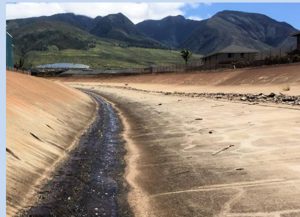
Stable concrete-lined stream channel at Kahoma Stream, Lahaina, Maui
