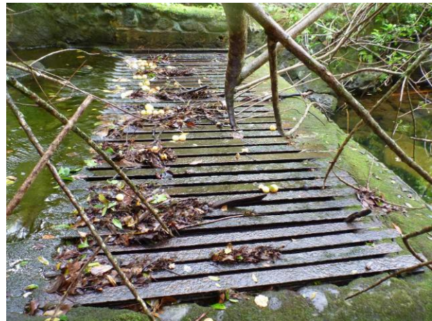
Honolua Stream diversion intake 769 from left bank (CWRM, 2011).
