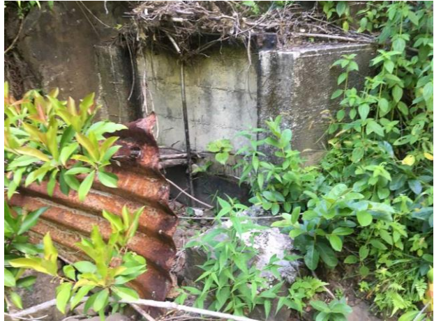
Close-up of intake control gate (CWRM, 2019)
