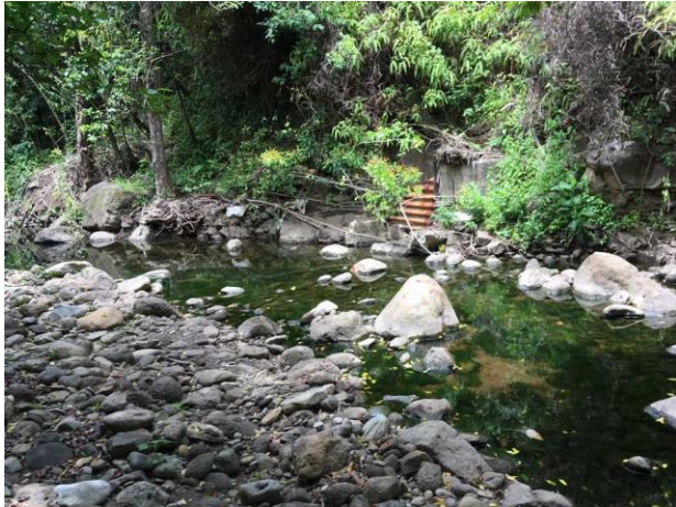
Honolua Stream from right bank, following hurricane damage in late 2018, with buried remnant diversion control gate on left bank (CWRM, 2019)
