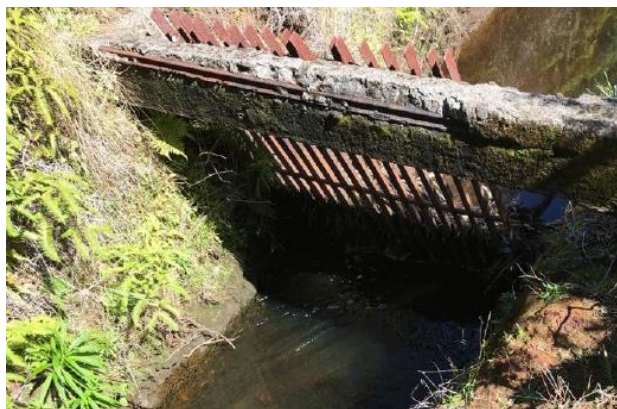
Trash rack and support beam at Waiakoali Ditch inlet (KIUC, 2020).
