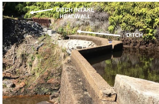
Diversion dam, looking toward ditch inlet and trash rack (KIUC, 2020).
