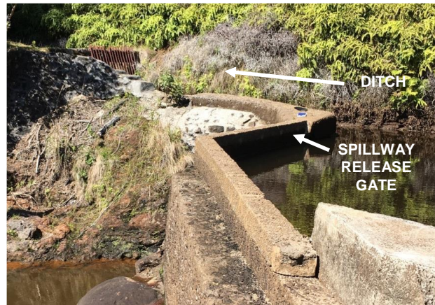
Diversion dam, looking toward ditch inlet and trash rack (KIUC, 2020).
