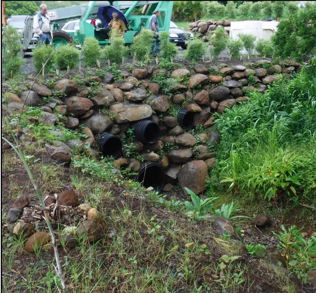
Remediation Area 5, mauka culvert looking downstream. (Staff July, 2017).
