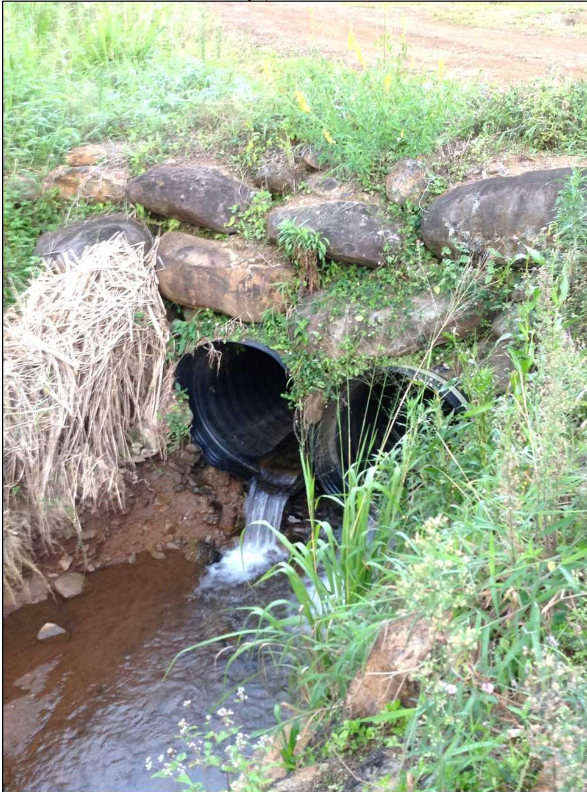
Remediation Area 2, makai culvert looking upstream. 2017.
