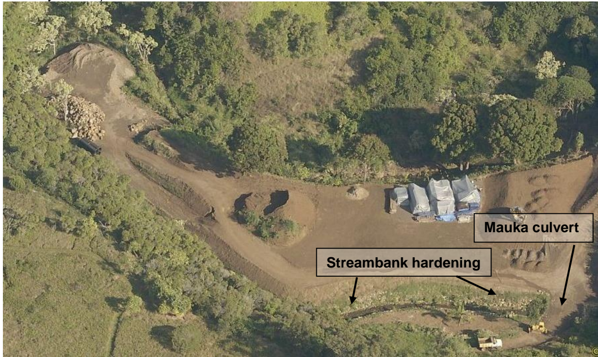
Remediation Area 5, streambank hardening below the mauka culvert looking makai. (Maui County website February 8, 2015).
