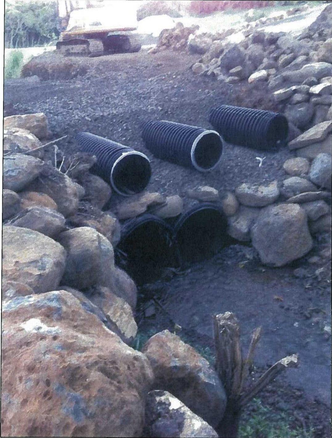
New culvert construction No. 1. Photo dated 2017.
