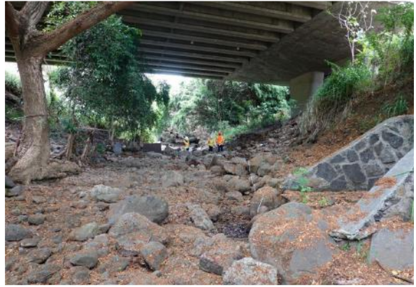
Figure 3: Looking downstream. Pier 26 on the right bank.
