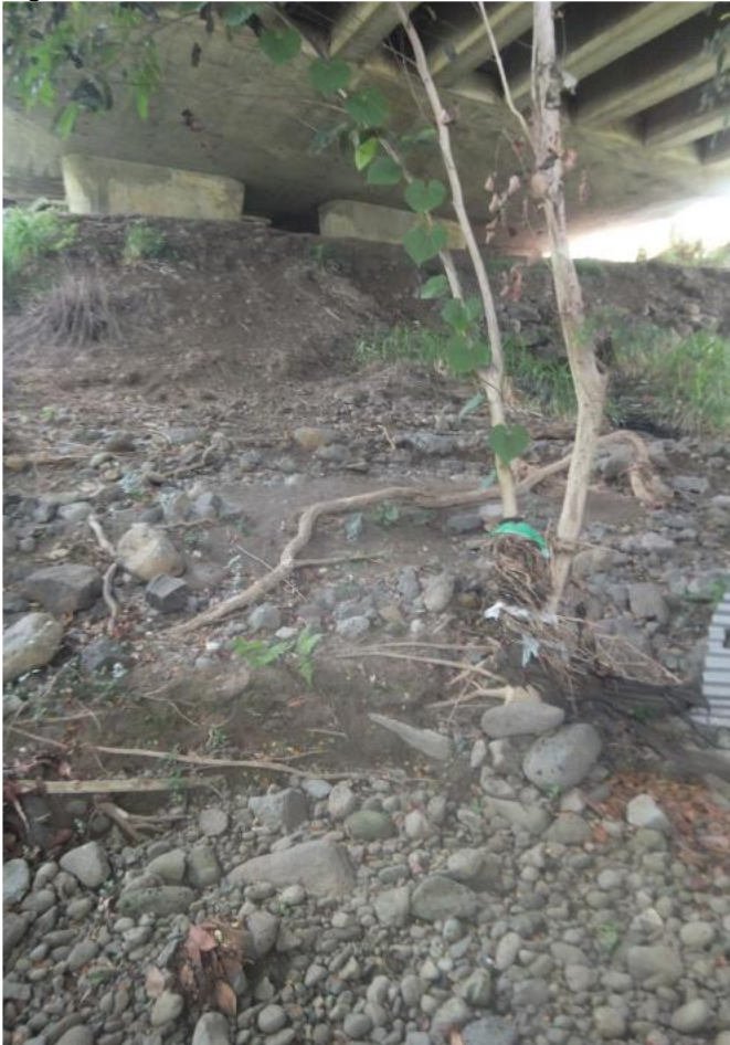
Figure 4: Pier 26, left bank.
