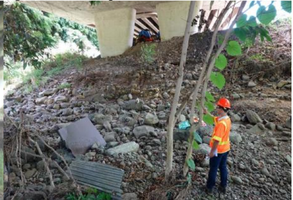
Figure 5: Pier 26, right bank.
