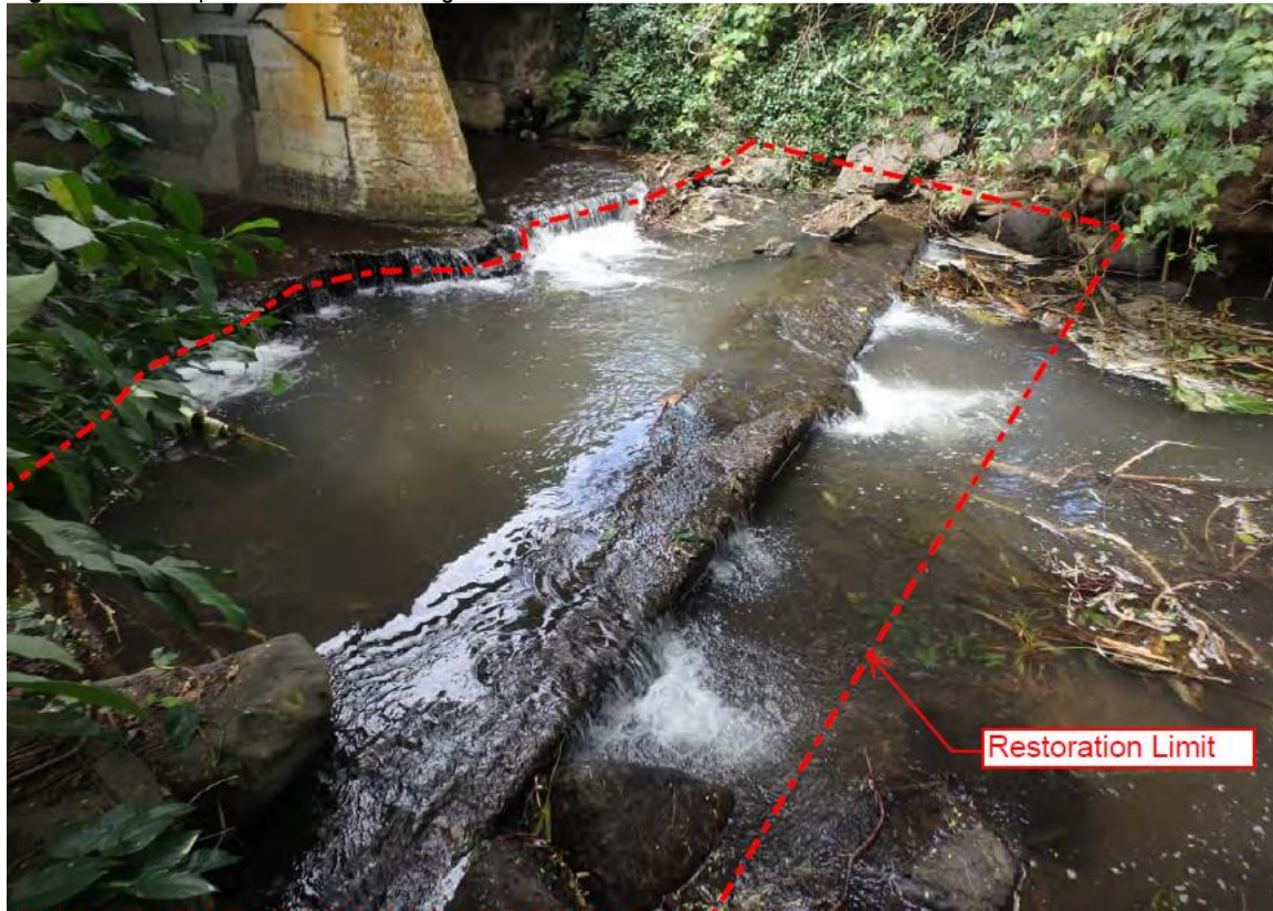
Figure 3: Close-up of force main crossing No. 1.
