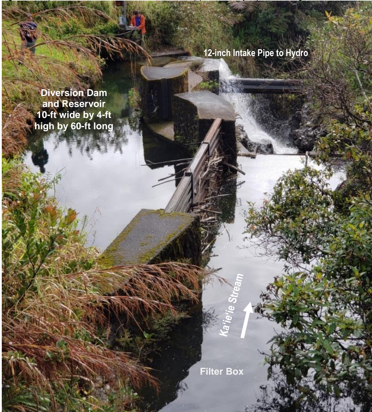
Figure 3: Site photos. Diversion dam, reservoir and 12-inch pipe intake to hydropower, looking downstream.
