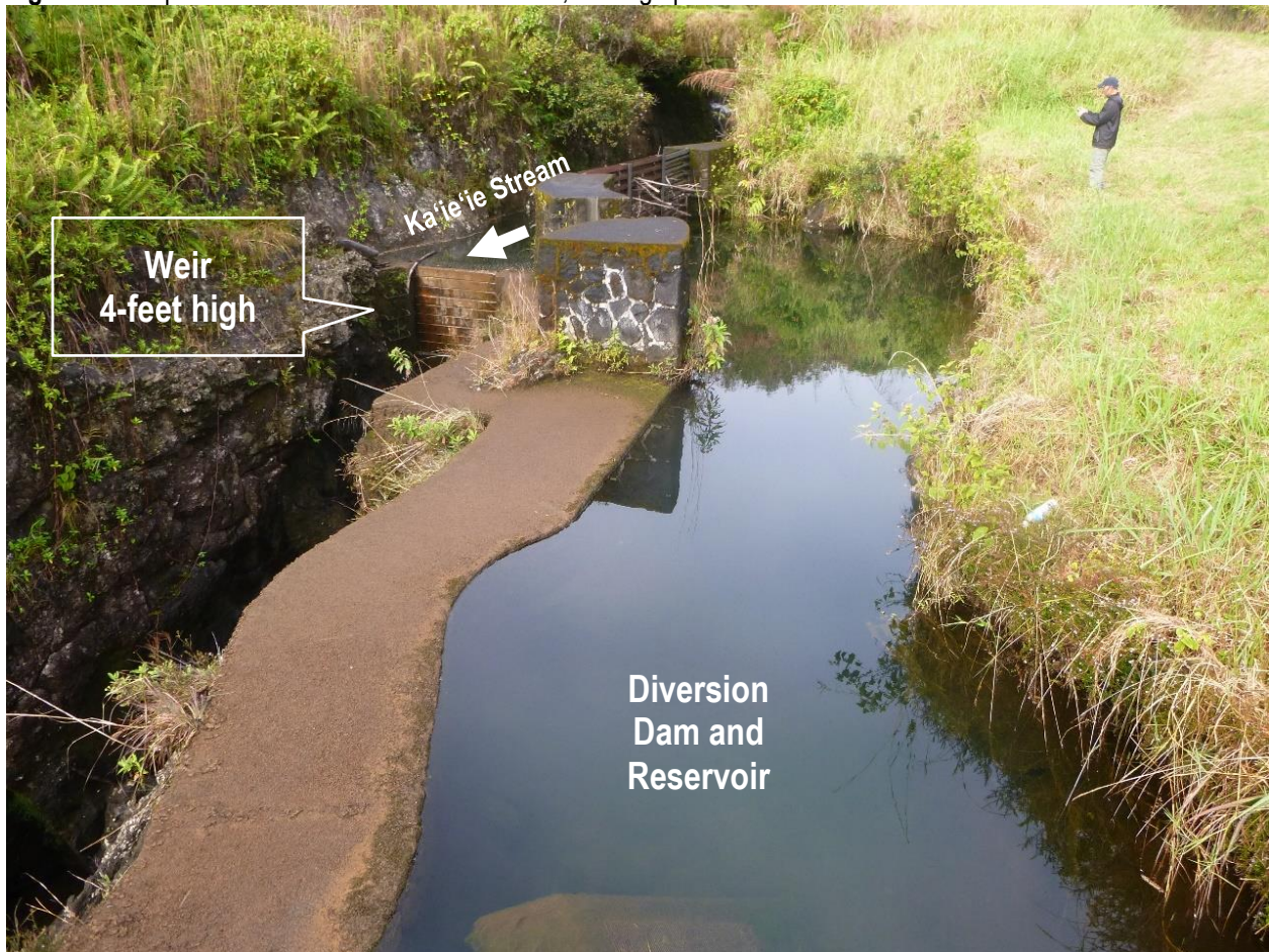
Diversion dam and weir, looking upstream. Reservoir is to the right.
