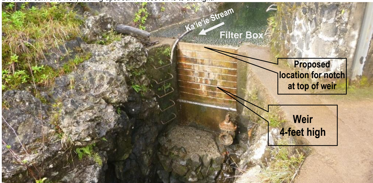
Diversion dam and weir, looking upstream. Reservoir is to the right.
