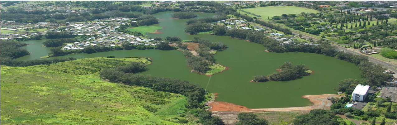
Aerial view of the basin and dam area of the reservoir.
