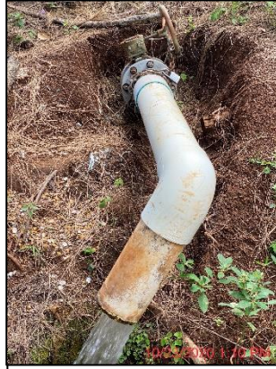
10-23-2020 (WWC Installed Valve & Lock)
