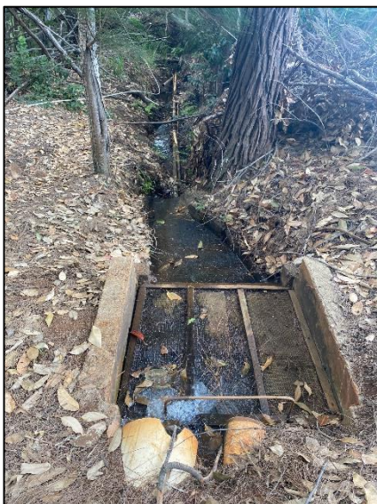
Clayton Suzuki private intake, water filtration system and pipeline within S. Waikapū Kuleana ‘Auwai 0.45 miles above downstream kuleana users and Native Hawaiian Kalo Farmers
