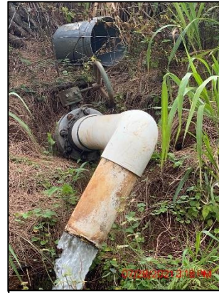
7-28-2021 (WWC Installed Valve & Lock)
