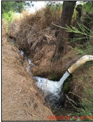
12-9-2019 (No WWC Valve and lock)
