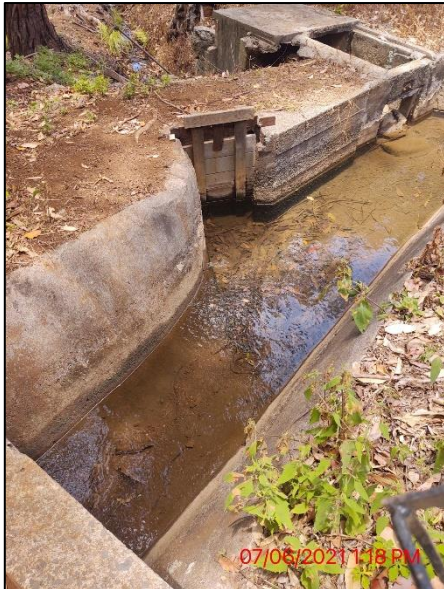
Sluice Gate immediately before Reservoir #1 that can flow directly into S. Waikapū kuleana ditch. Refer to Exhibit A for explicit location on schematic map.
