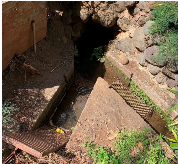
19) Water flows from a driveway culvert at the Velez (Higa) property and splits. The right channel goes towards Velez and Ciotti (Velez pulls water from the channel via a pipe). The left channel continues towards the Ibara property.
