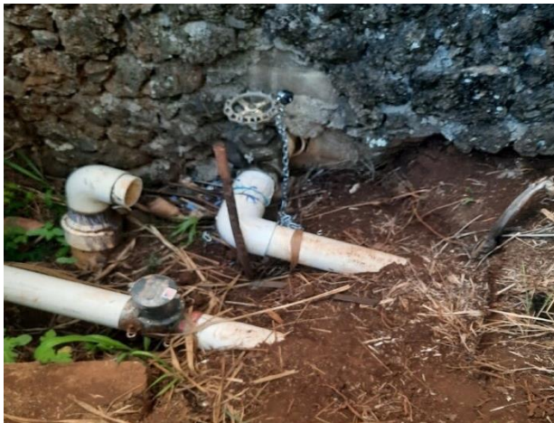
6) Cut chain on distribution pipe valve to the Wailuku Town Kuleana ‘Auwai on October 25, 2021.
