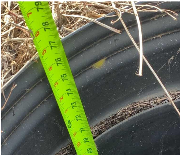
24) Measured depth (approx. 6'6") from ground surface to the bottom of Waihe'e Ditch where the control valve is located.
