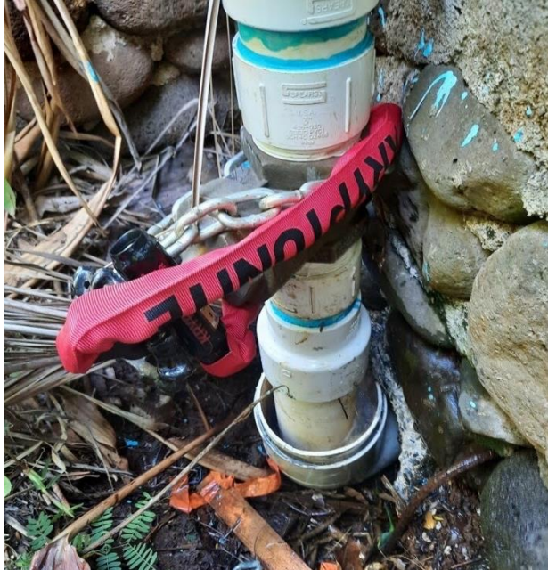
26) Kryptonite lock installed on the Wailuku Town Kuleana 'Auwai distribution pipe.
