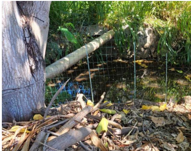
23) Excess water flows through a pipe at the edge of the Ciotti property into Spreckels Ditch.
