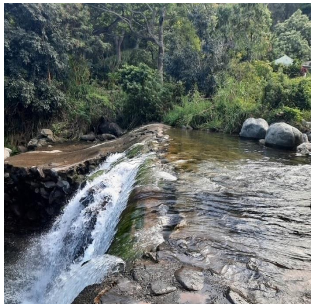
33) Wailuku River following repair of the Siphon, at center.
