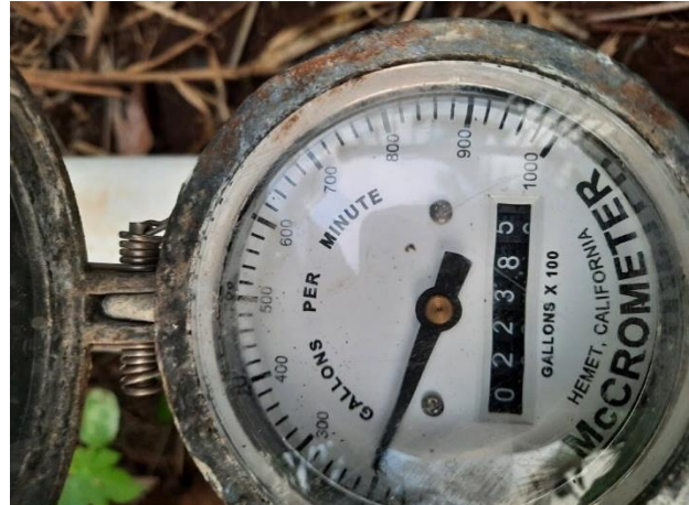
5) Flow meter on the distribution pipe to the Wailuku Town Kuleana 'Auwai. Reading indicates slightly more than 100 gpm, and a total of 2,238,500 gallons.
