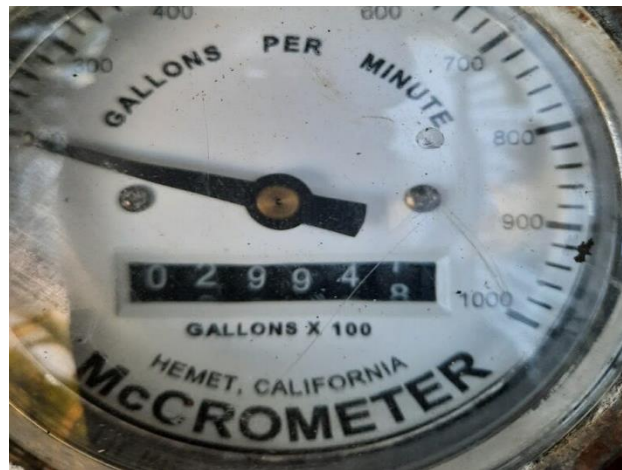
7) Flow meter on the distribution pipe to the Wailuku Town Kuleana ‘Auwai. Reading indicates approx. 200 gpm, and a total reading of 2,994,800 gallons.
