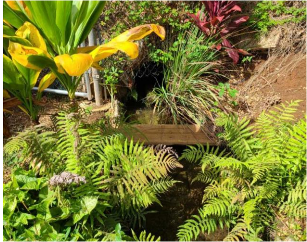
9) Water flows underground from Imua Family Services and drops into an open ditch on the Koeli LLC property.
