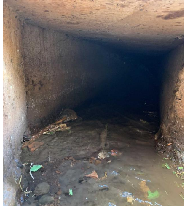
13) Water flow in underground concrete-lined channel behind Wailuku Public Library.
