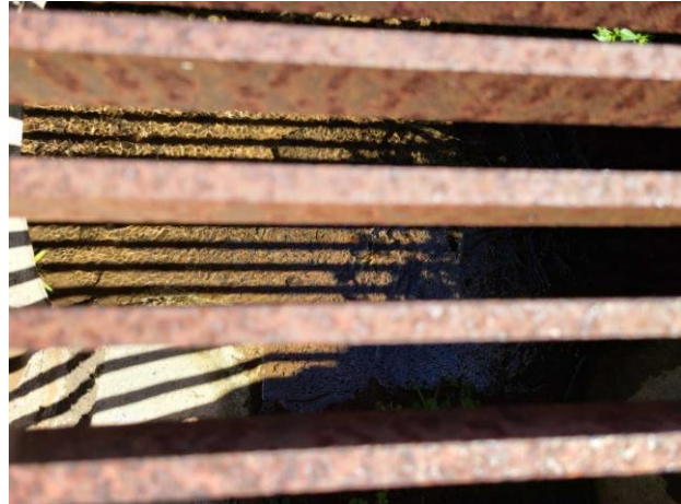
17) Close-up of water flowing ditch at 436 Kalua Road.
