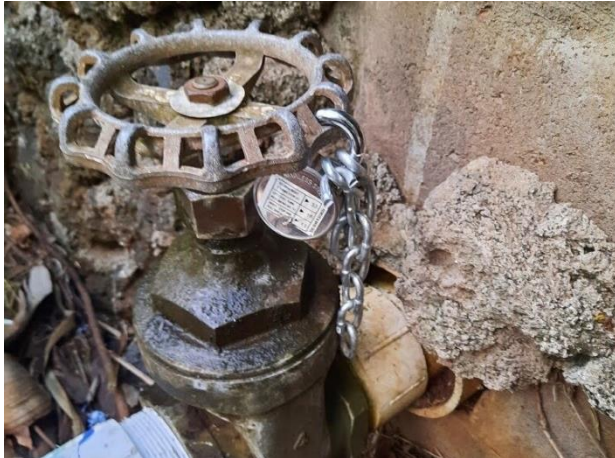
4) Cut chain on distribution pipe valve to the Wailuku Town Kuleana 'Auwai.
