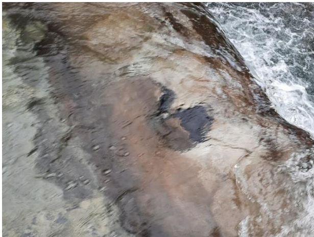
30) Ruptured siphon at Wailuku River.
