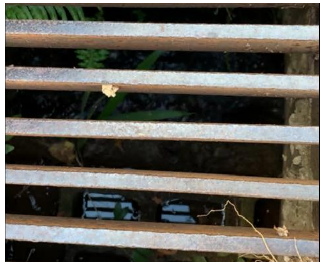
15) Close-up of water flowing in concrete-lined channel approximately six (6) feet underground.
