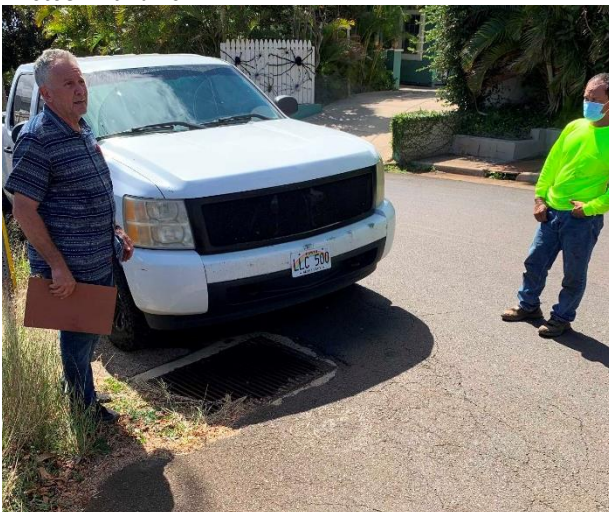
14) Storm drain grate at the corner of Kaohu Street and Kalua Road, where channel continues underground towards the left of the photo along Kalua Road.
