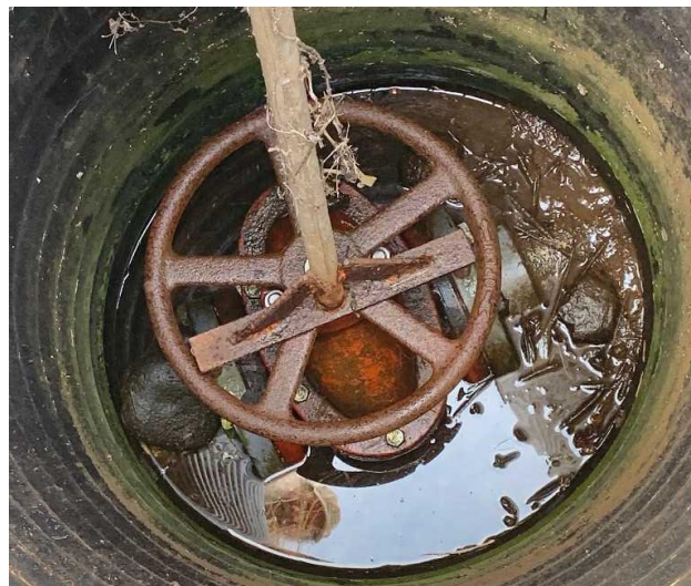
25) Control valve for the intake pipe located on Waihe'e Ditch which feeds the distribution pipe to the Wailuku Town Kuleana 'Auwai.
