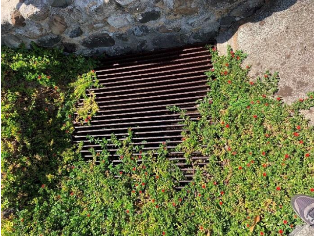
16) Storm drain at 436 Kalua Road.
