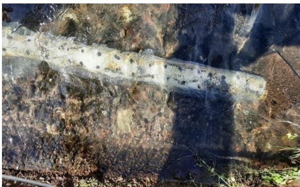
3) Perforated screen installed on intake pipe at Waihe'e Ditch.
