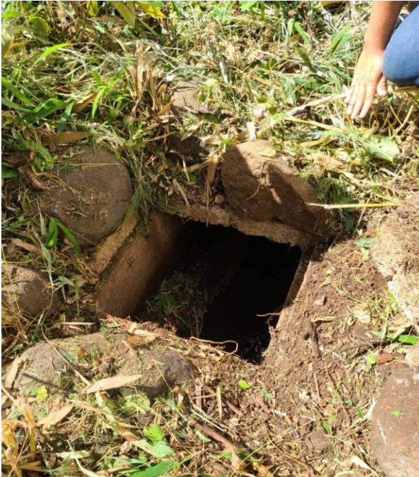
12) Uncovered access point of underground concrete-lined channel behind Wailuku Public Library.
