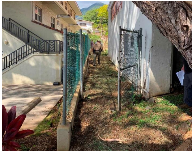
11) The access gate behind the Wailuku Public Library to observe the access point on the underground concrete-lined channel.
