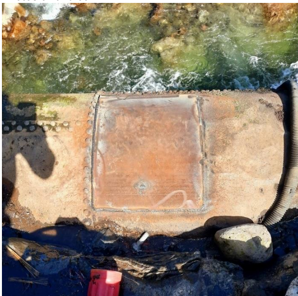
32) Repaired siphon at Wailuku River.
