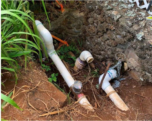
8) Distribution pipe with valve chained and flow meter at center, located on the boundary of Imua Family Services property.
