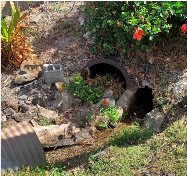
18) Water exits underground pipe and flows into an unlined channel and enters a culvert under a driveway.
