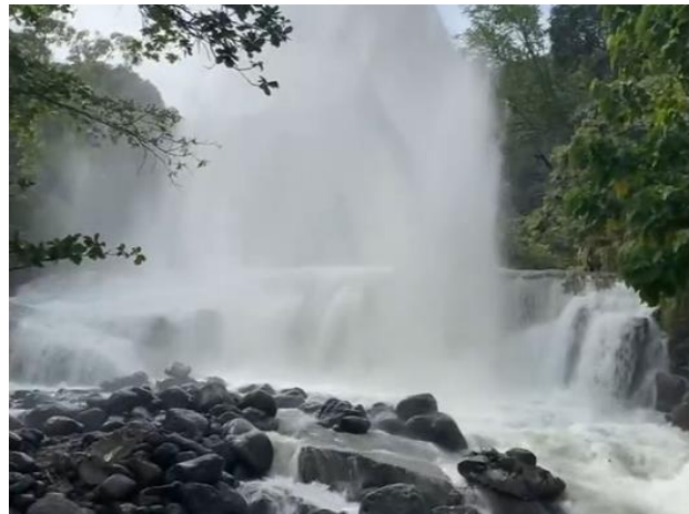
31) Screenshot of damaged siphon from Hawaii News Now newscast on December 10, 2021. Recording was provided courtesy of Hui o Nā Wai ‘Ehā.
