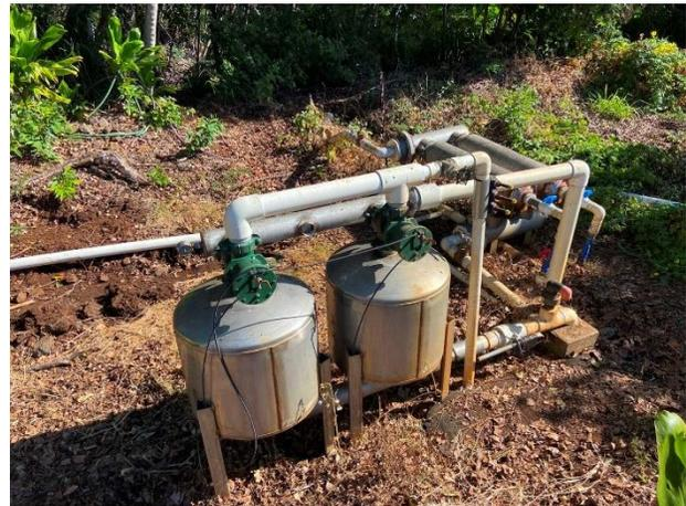
14) Mr. Suzuki's sand filters with lateral (at left) from 4-inch lateral line, awaiting connection.
