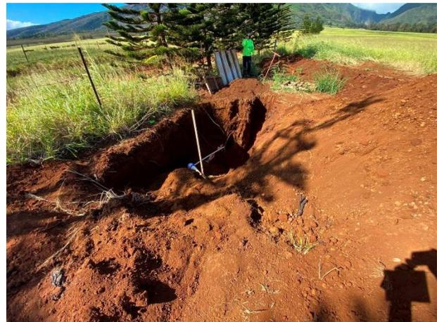
12) Installation of lateral 4-inch line off of main 8-inch line.
