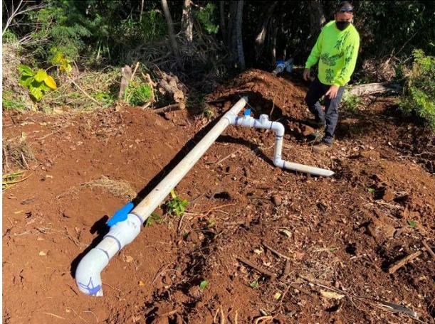
15) Lateral 4-inch line, with line to Suzuki at left, then continues to South Waikapū Kuleana ‘Auwai in background. Meter will be installed after the ball (control) valve in the foreground.
