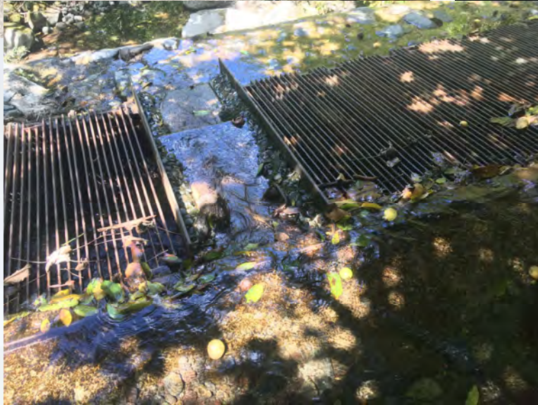
Plate on Dam #1
