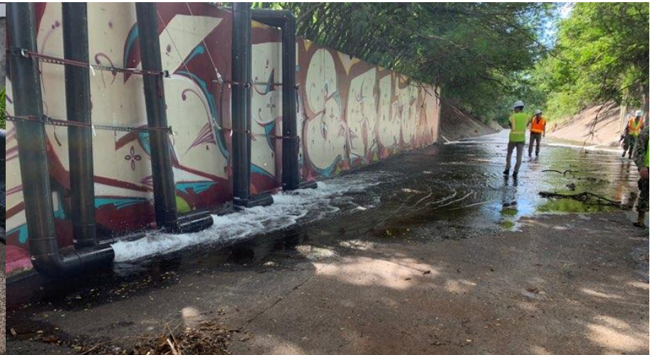
Monitoring 5MGD GAC Discharge
