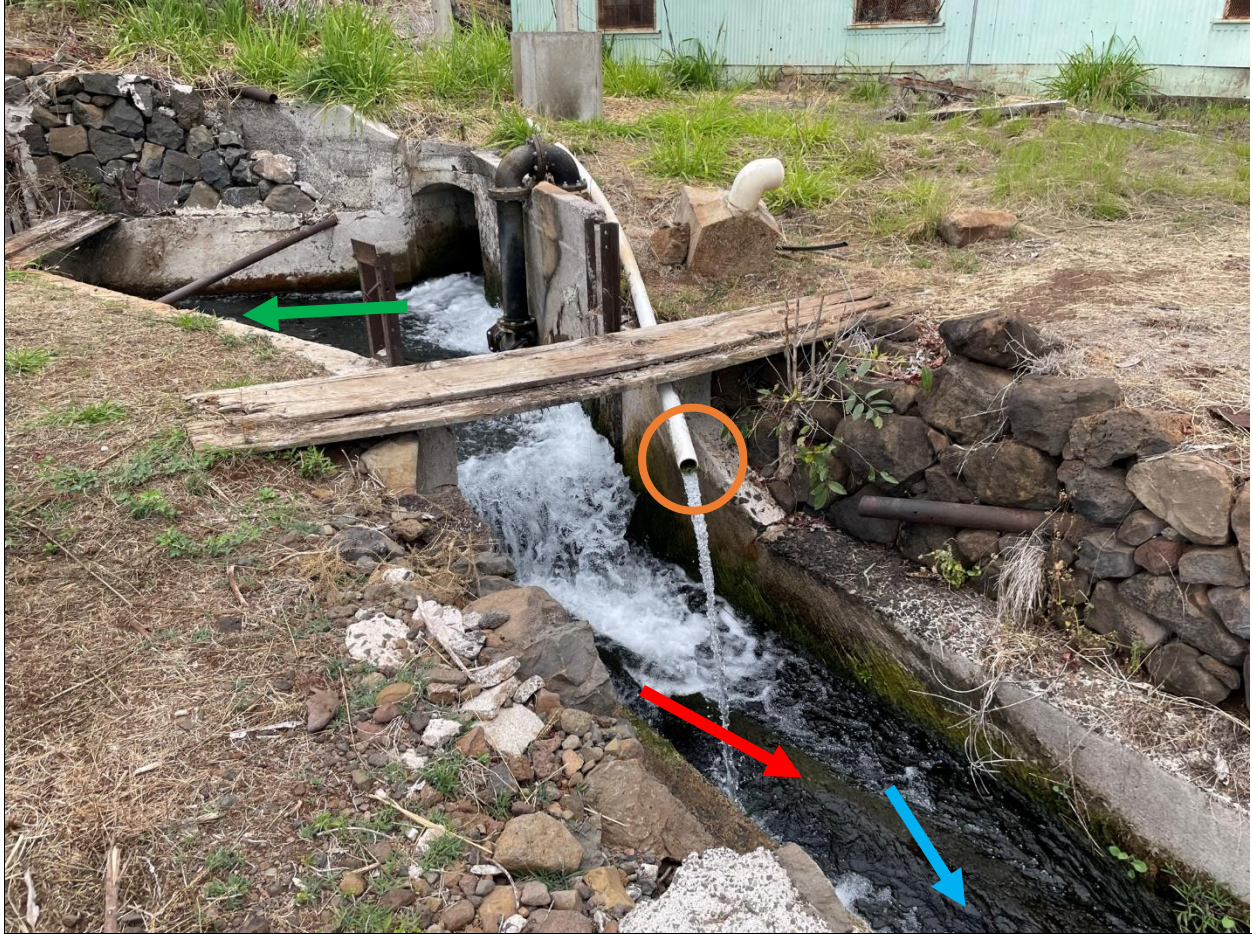
Figure 4. Kaua'ula Ditch below the hydropower tailrace. Flow of water to Kamehameha Schools tenants is indicated by the green arrow (water is conveyed in a pipeline located in the ditch, with its intake situated further upstream in the tailrace tunnel to the right), return flow from lo'i complex mauka of hydropower plant indicated in orange circle, pipeline to Kuleana families in valley is indicated by the red arrow (water is conveyed in a pipeline located in the ditch), and downstream direction of flow in ditch to siphon indicated by the blue arrow.
