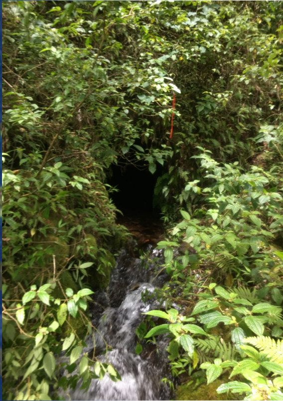
Tunnel 22 Honokōhau Gulch Honokōhau hydrologic unit
