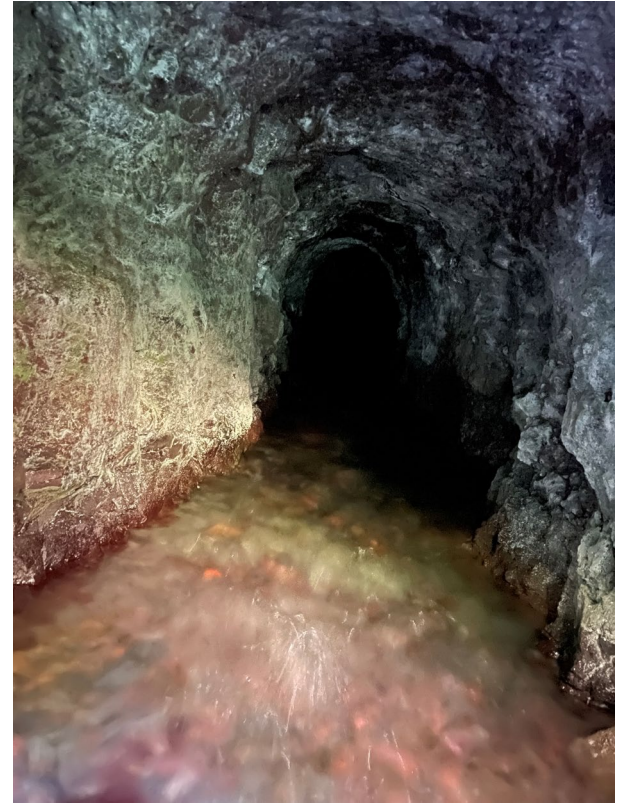
Tunnel 18 Kahoma Valley Launiupoko hydrologic unit
