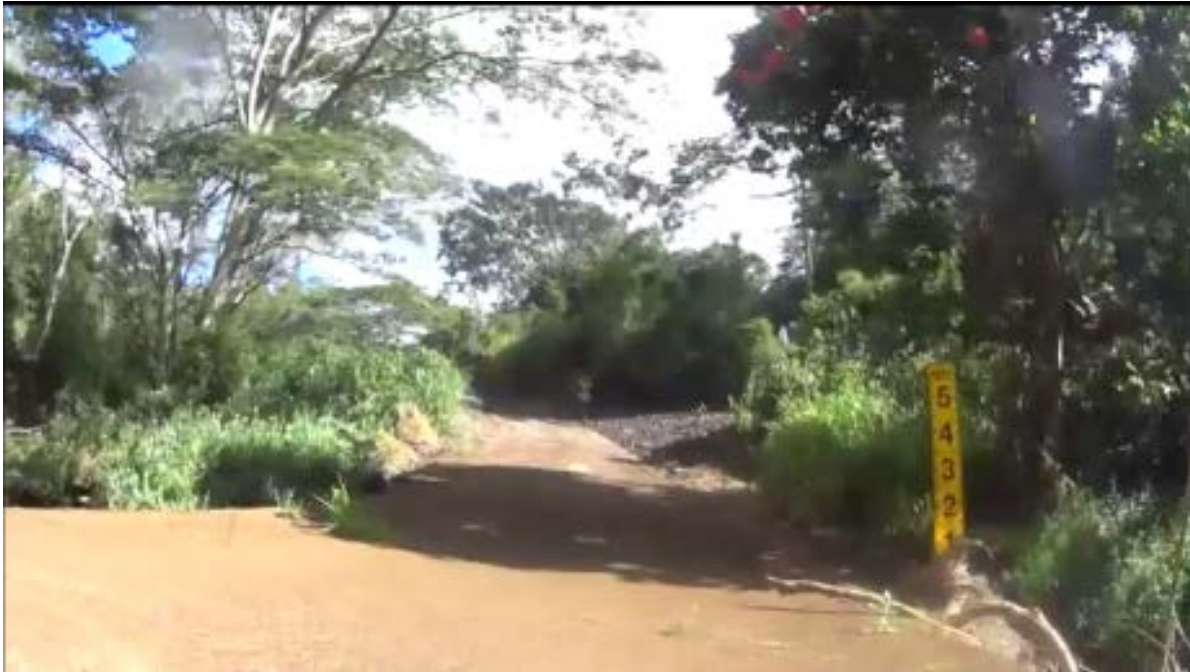
Figure 1. Site 1 stream road crossing below the reservoir. Note water level gauge on the right side of the road.
