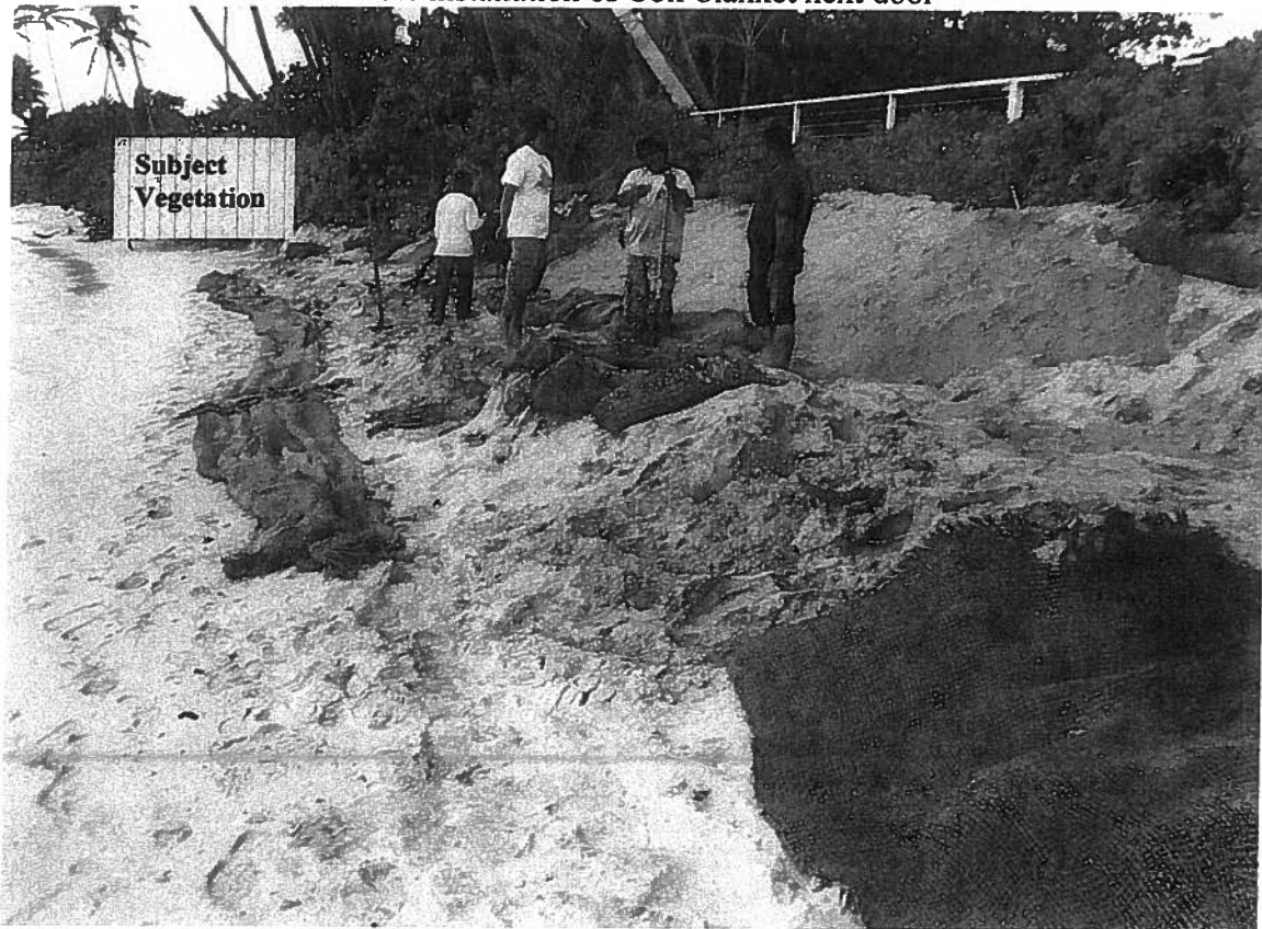
Site Photo December 11, 2009 Note installation of Coir blanket next door
