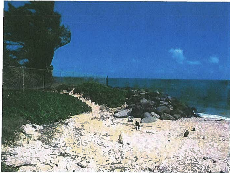
East Flank of Existing Revetment
