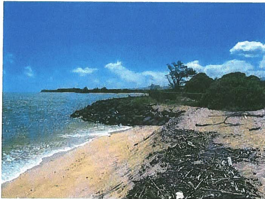
West Flank of Existing Revetment
