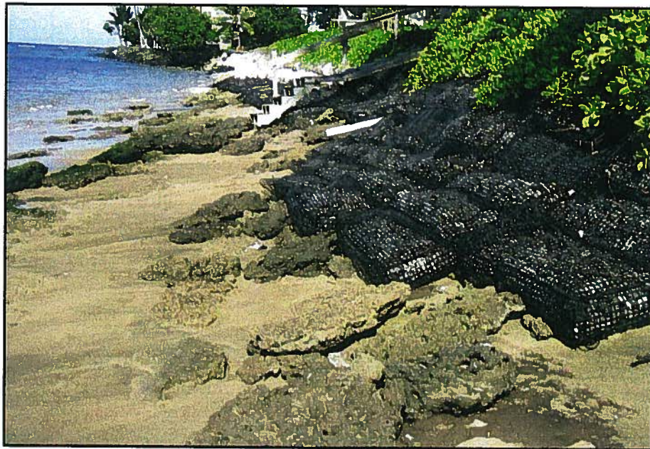
Beach rock fragments exposed during low sand conditions; note draped rock mattress shore protection at adjoining Royal Kahana property
