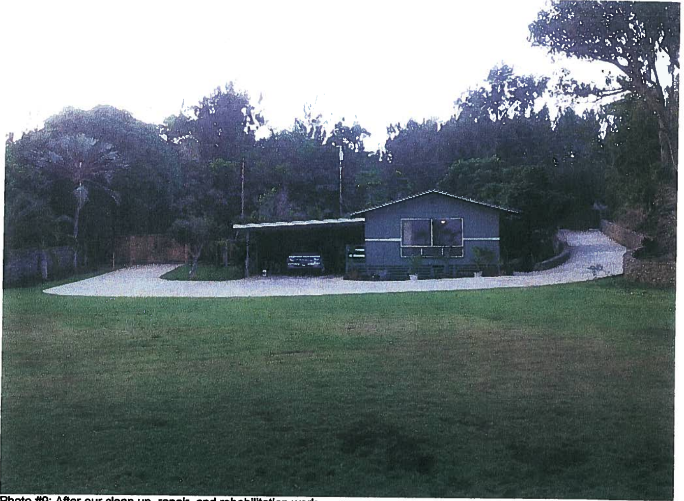
Photo #9: After our clean up, repair, and rehabilitation work
