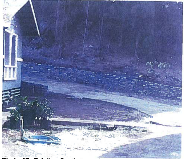
Photo #5: Existing Southern rock walls before repair.
