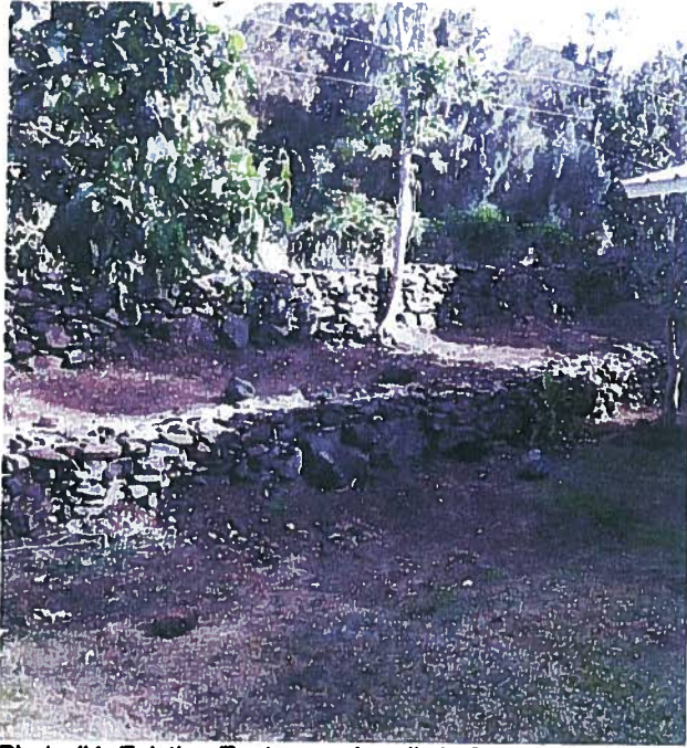
Photo #4: Existing Eastern rock walls before repair.
