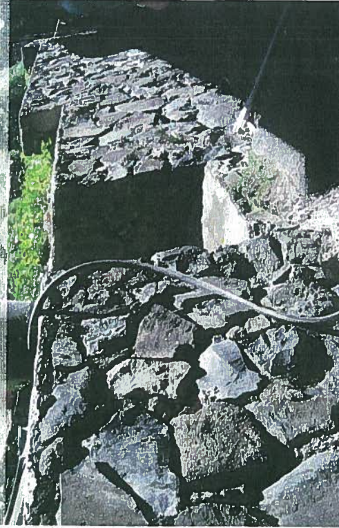
EARTH RETENTION STRUCTURE PARALLEL TO GUEST RESIDENCE
