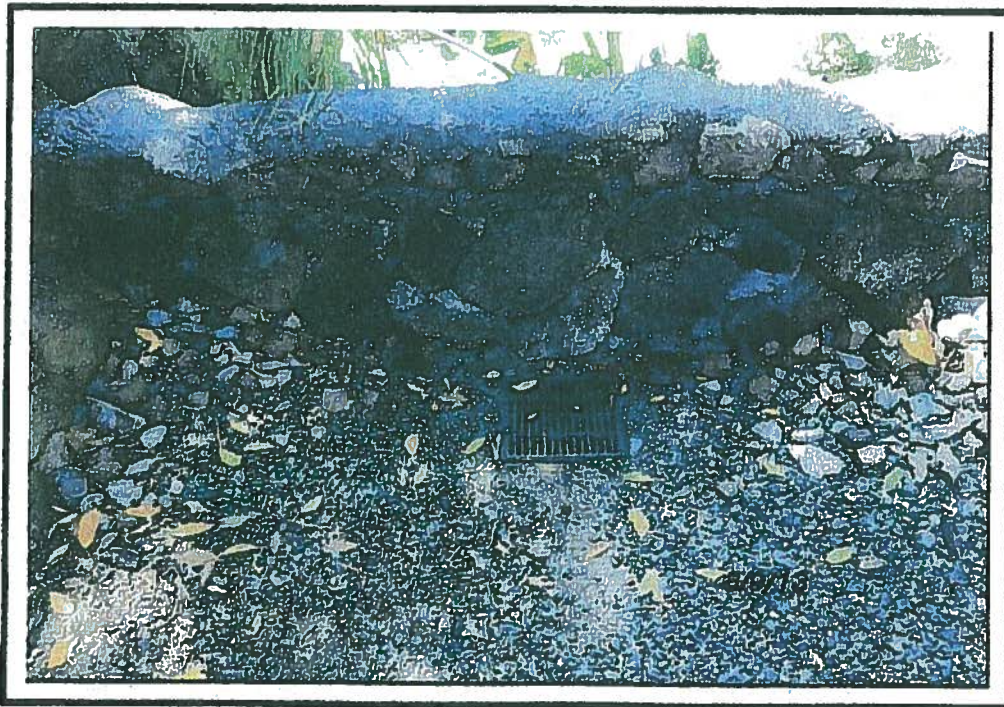
At dam, looking down toward CRM wall and drain inlet.
