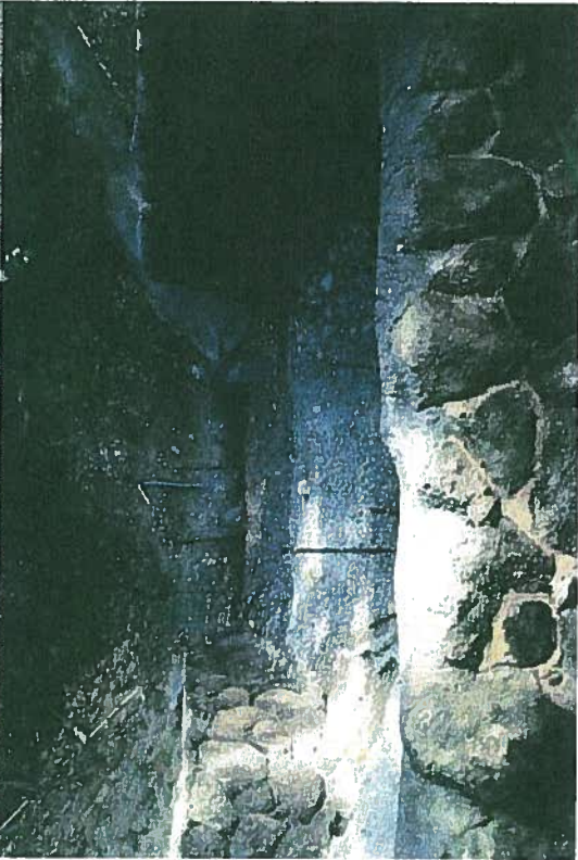
EARTH RETENTION WALLS NEAR MAIN RESIDENCE
