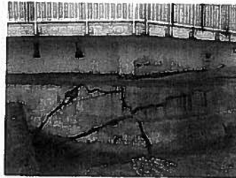
Cracks have increased in size since 21 DEC 2008, indicating continued erosion and settling. Clear loss of sand is evidenced.
