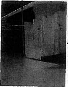
① CONCRETE WALL SITE AND TILE WALL
