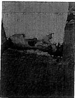
B-2.1 WALL DAMAGE
