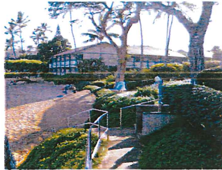
Install public shower signage
