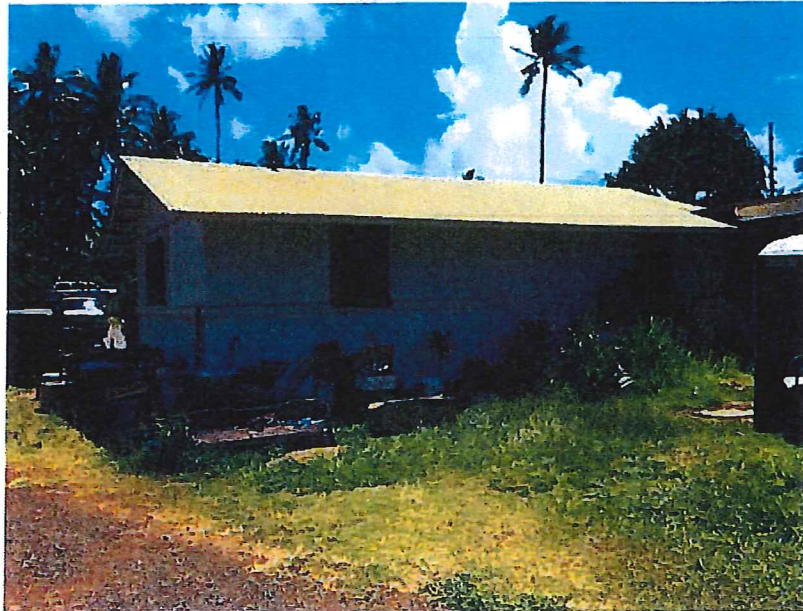
Elevation facing northeast
