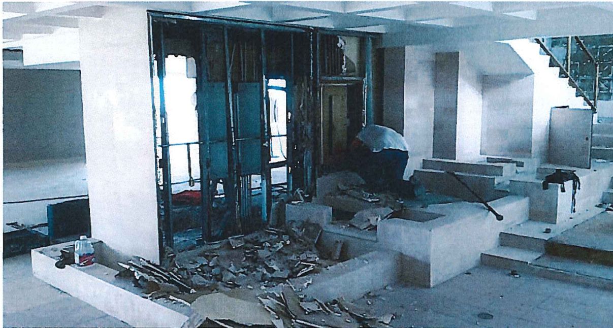
Lower wall, stair, and water feature demolition
