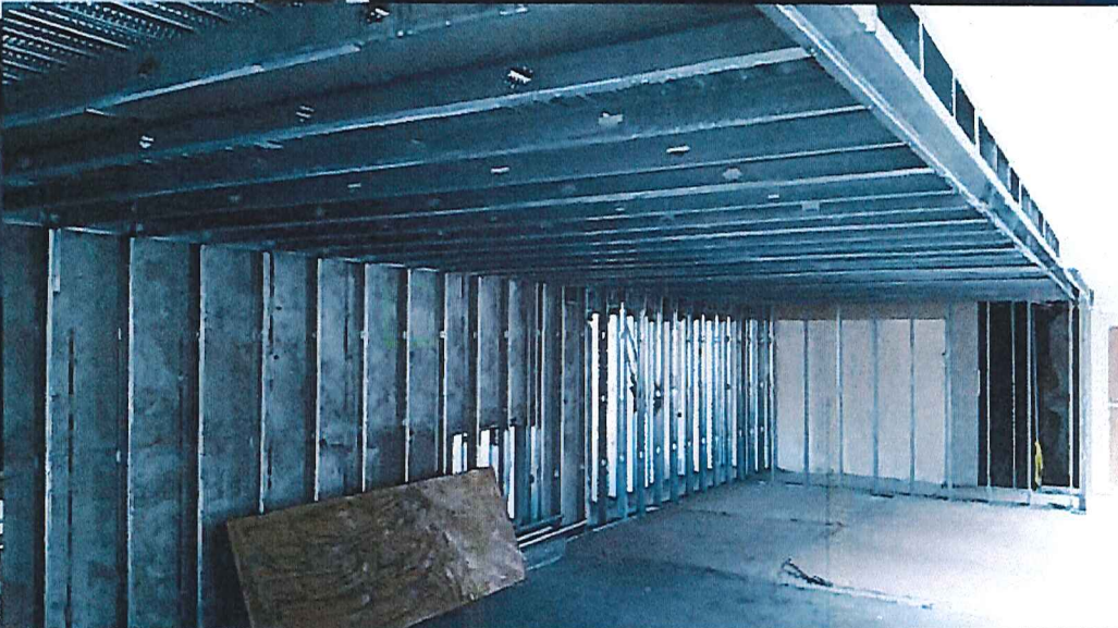
Lower level game room wall and ceiling framing and preparation for sprinkler installation
