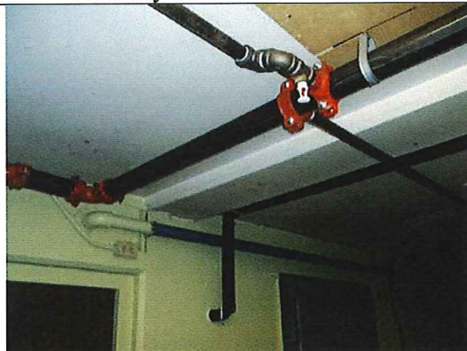
New Fire Sprinkler System
