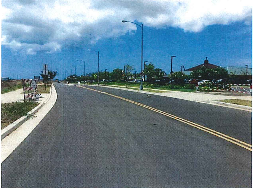
Photo (dtd April 22, 2015) of Road E looking southwest. KROC Center is on the right.
