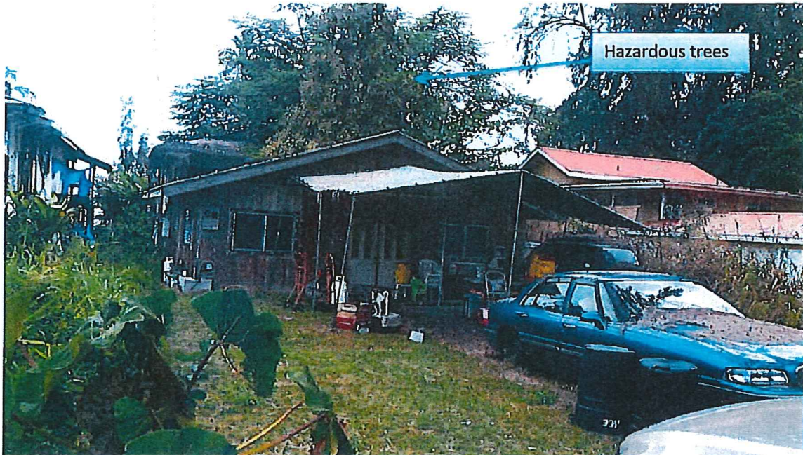
View from street – note overgrown trees on roof. Two inoperable vehicles sitting in front yard area.
