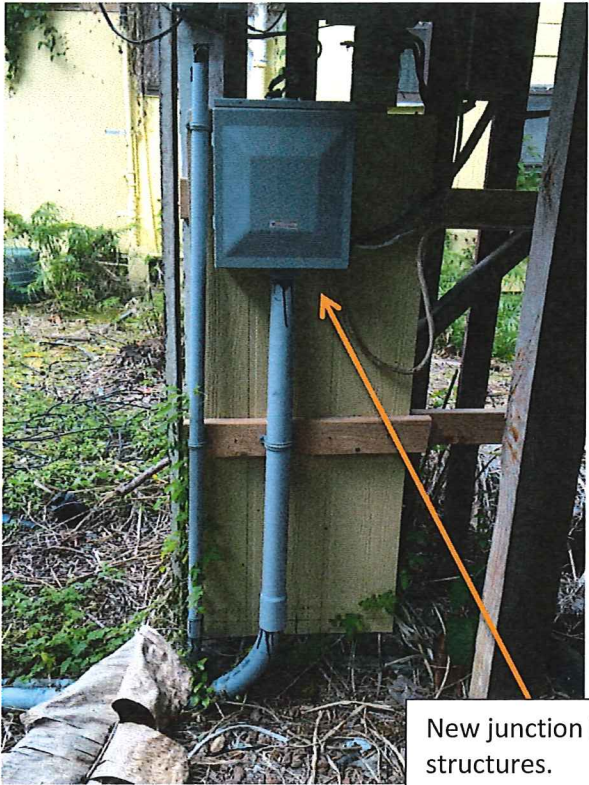
Conduit between boxes crosses wastewater pipe.
