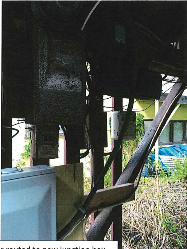
Original service panel with jumper routed to new junction box.
