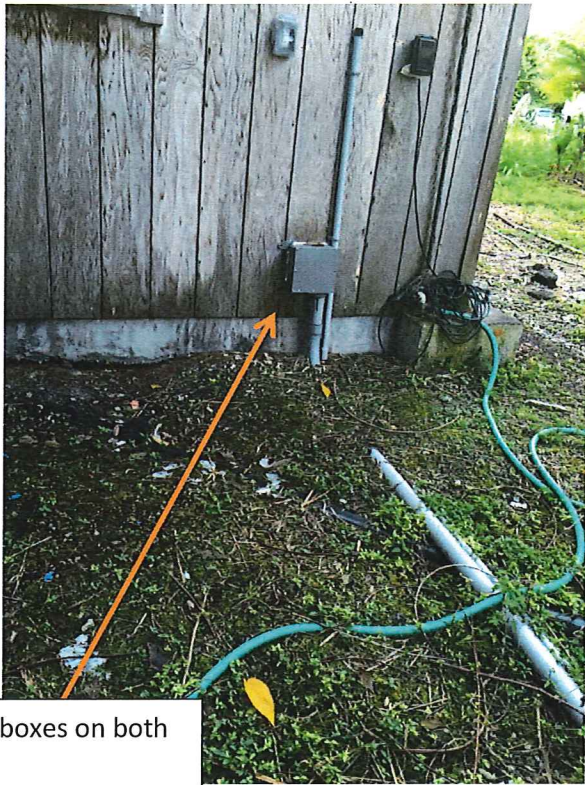
Conduit between boxes crosses wastewater pipe.
