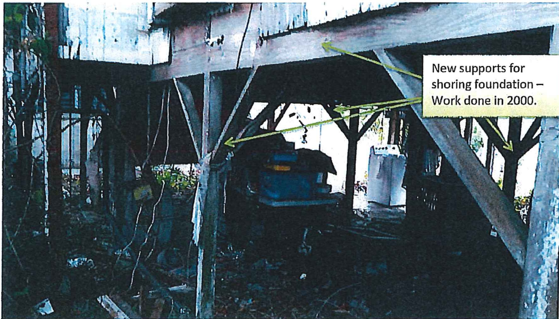
View of underneath of original house. The debris, wiring and vines are representative of overall condition of premises.
