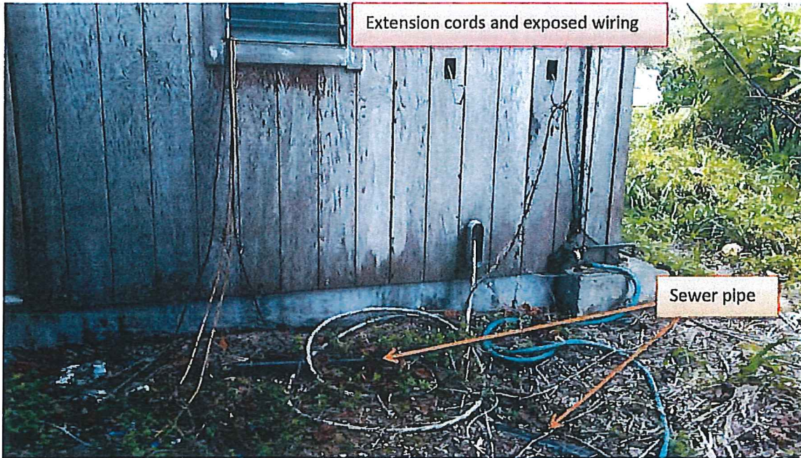
Area at rear of garage – between the two structures. Note black sewer pipe from garage structure.
