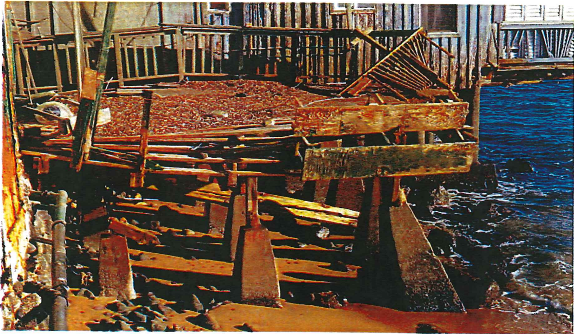
Deck and piers when viewed from access hallway
