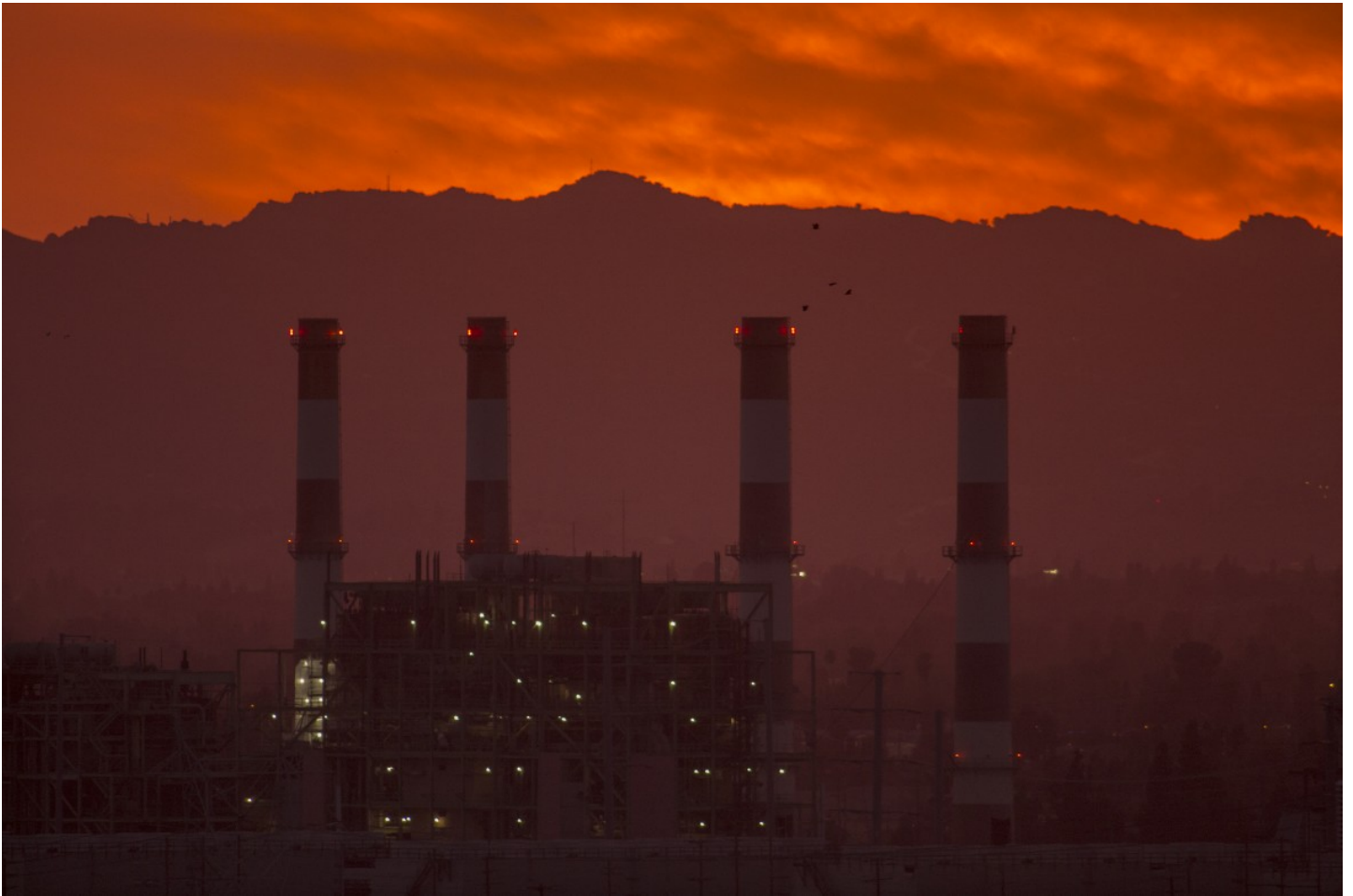
A gas-powered plant operating in California's San Fernando Valley.
