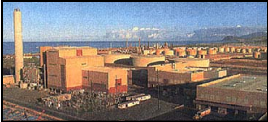
Photo 3.1 City and County of Honolulu's H-POWER
