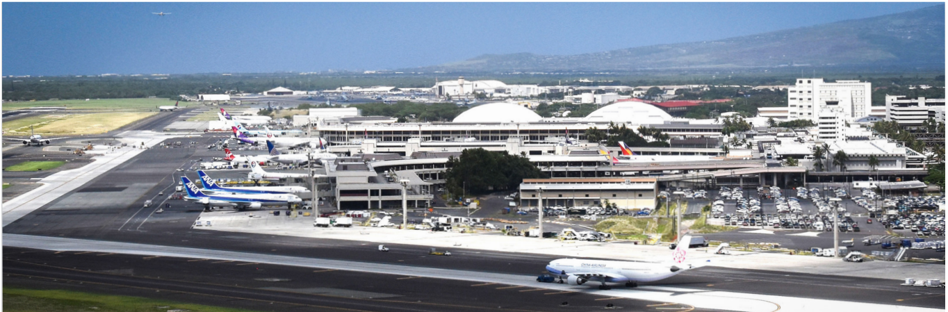
PHOTO: HAWAII DOT AIRPORTS DIVISION
