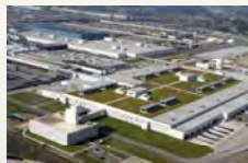
The Ford Motor Company assembly plant in Dearborn, MI The green roof covers 10.4 acres
