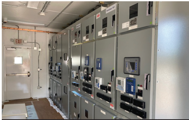
PEARL microgrid's Power Distribution Center; the control room for utility and cyber security systems
