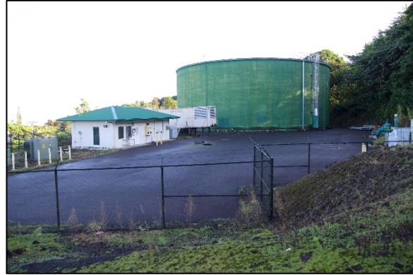
View northwest toward the existing Wai‘aha Well and Reservoir.
