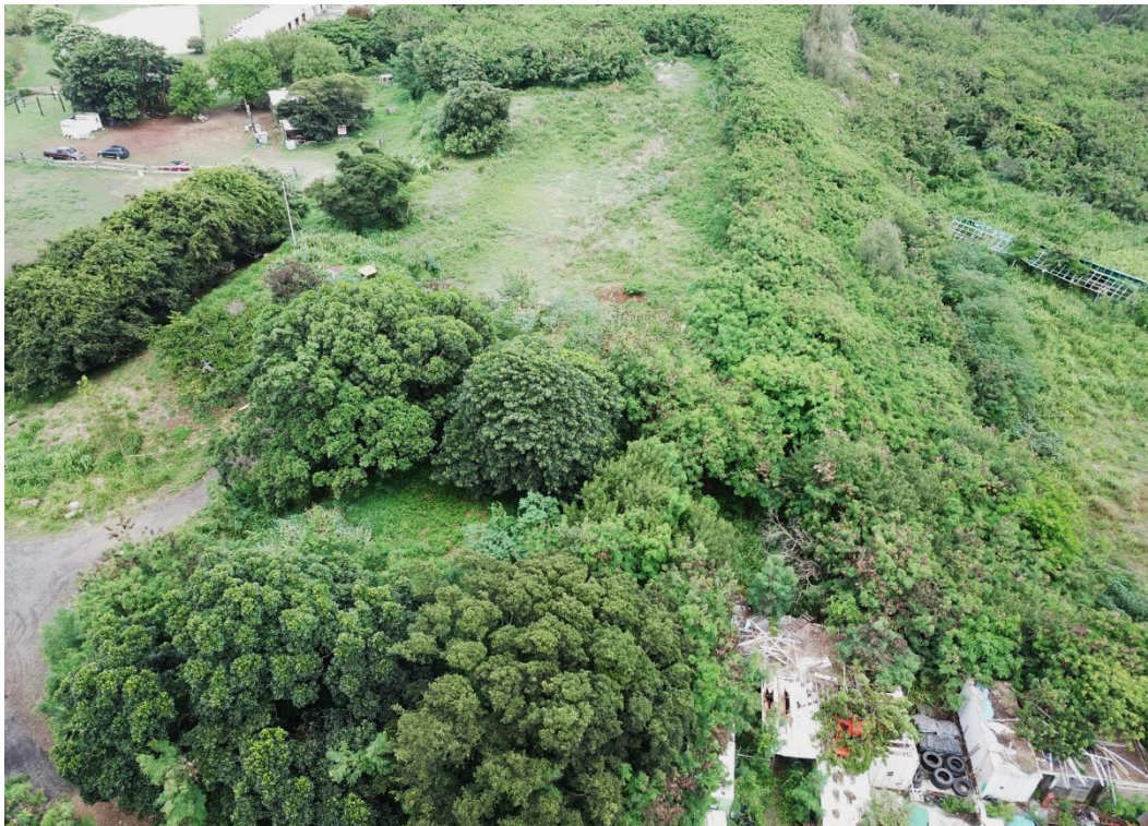
Photo #10 Overview of existing equestrian facilities, storage uses and solid waste concerns including an abandoned steel-framed structure (near upper right corner of photograph) within the southern portion of the project site.
