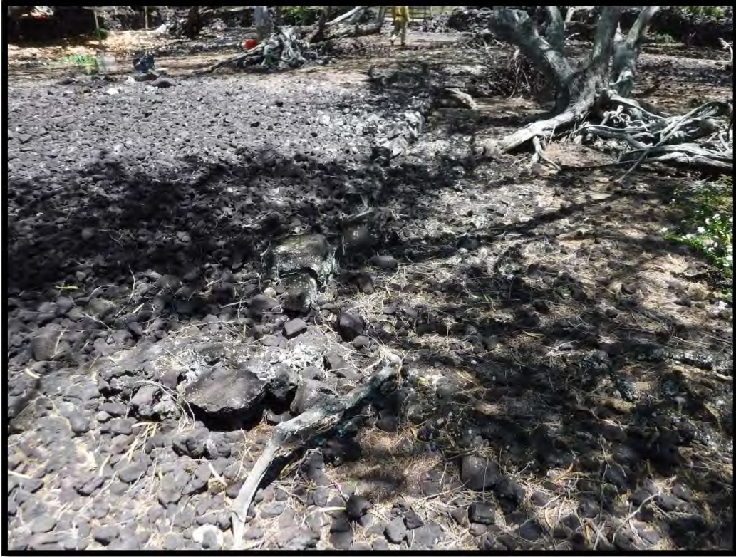
Figure 16. Retaining wall along south side of Feature A terrace (view to east-northeast)
