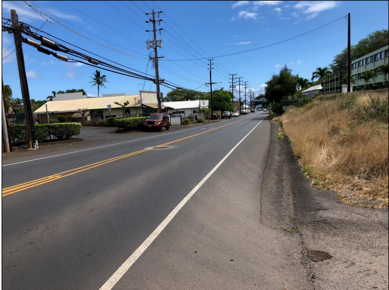
Figure 6. General view from the southwestern end of the project area (nearest Ainahou Place) showing the built environment and an existing sewer manhole in the center of Lower Main Street, view to northeast
