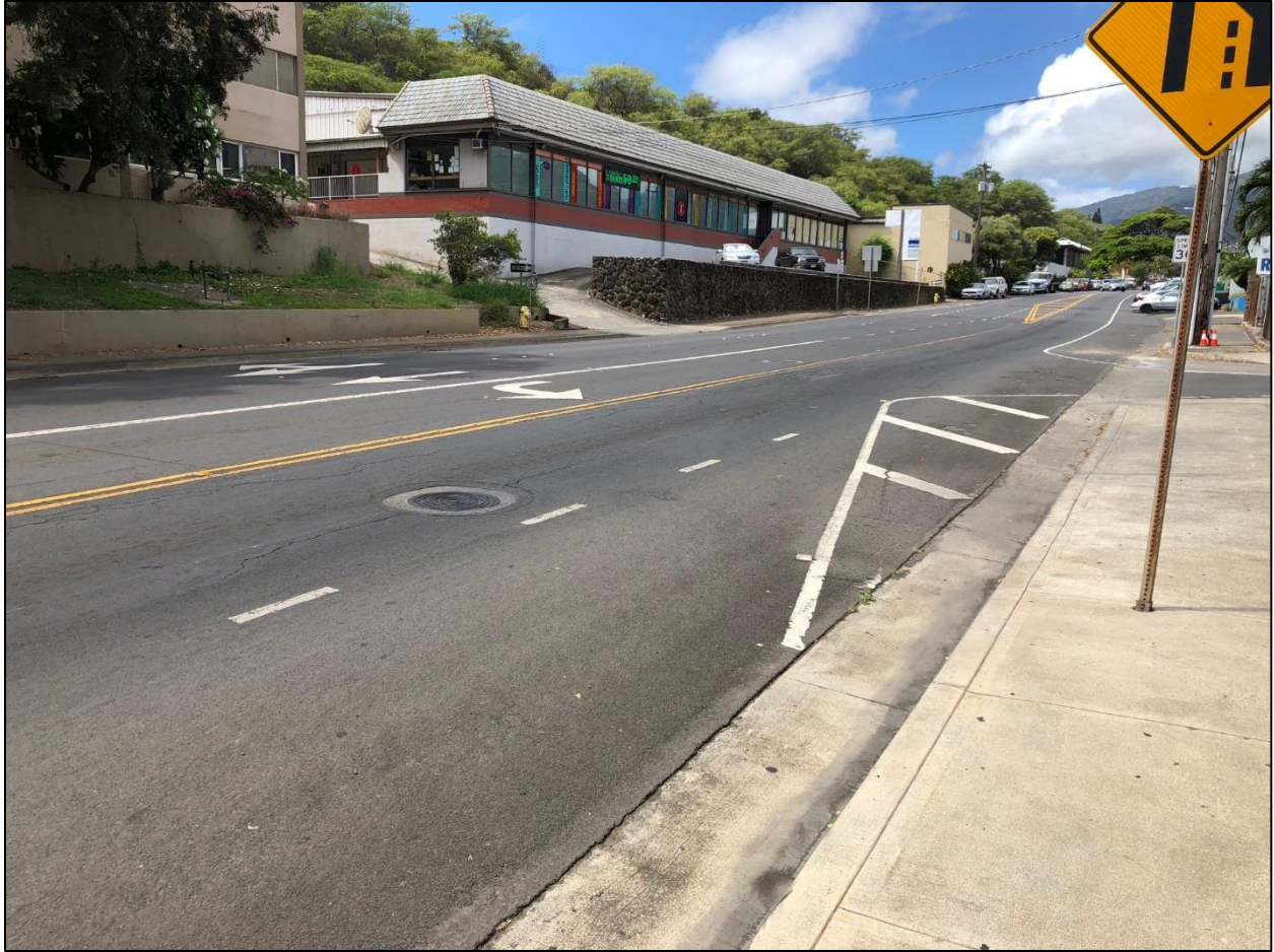
Figure 7. General view from the northeastern end of the project area (nearest Waena Street) showing the built environment and an existing sewer manhole in the center of Lower Main Street, view to southwest
