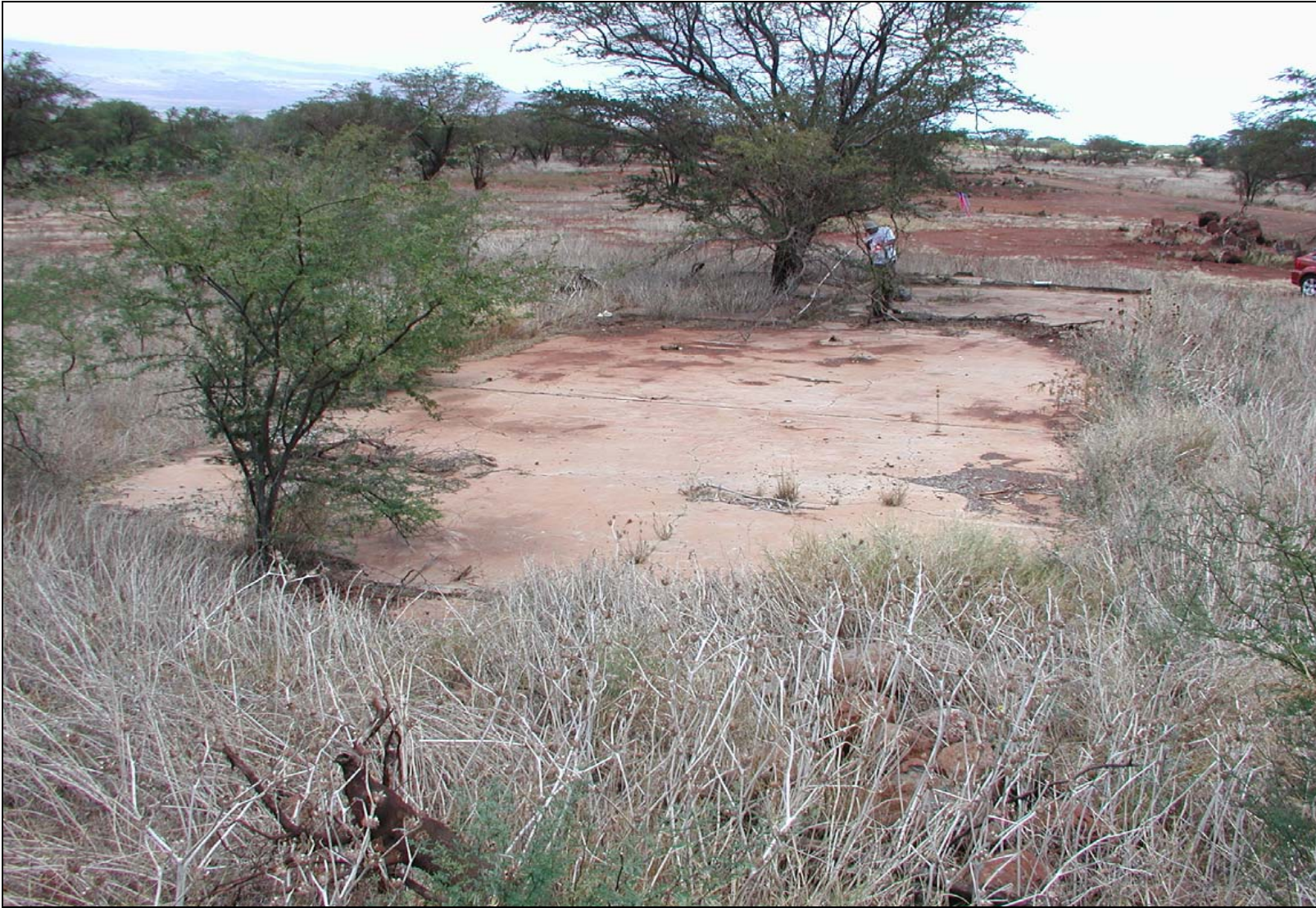
Figure 10: Photograph of SCS Site T-14 Foundation Over View. View to Southeast.
