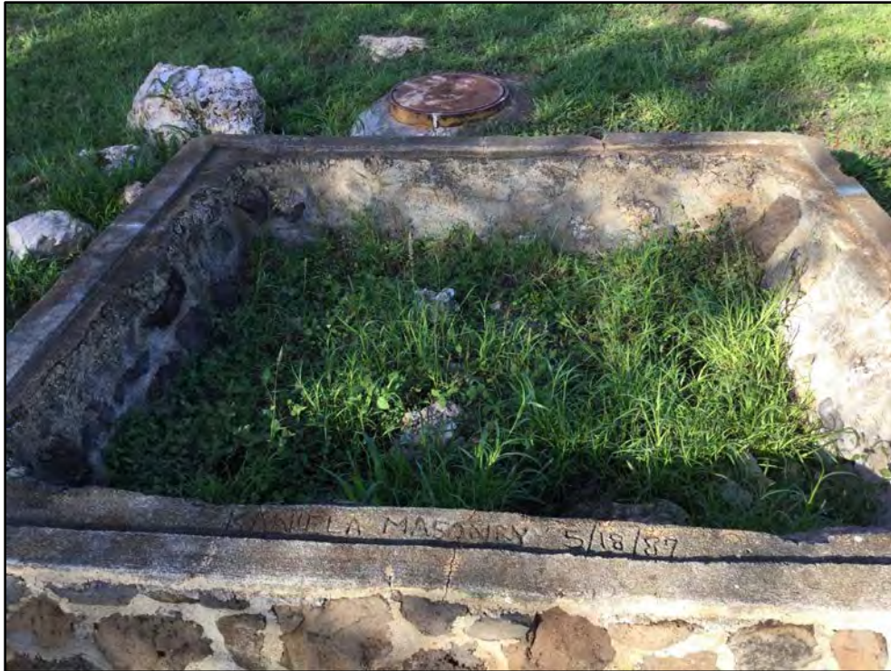
Figure 89. Basalt and concrete mortar planter along Wākea Street, note the engraving saying “KANIELA MASONRY 5/18/87,” view to west
