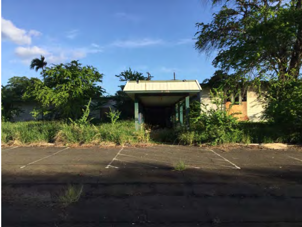
Figure 97. Abandoned buildings along Road A segment, view to north
