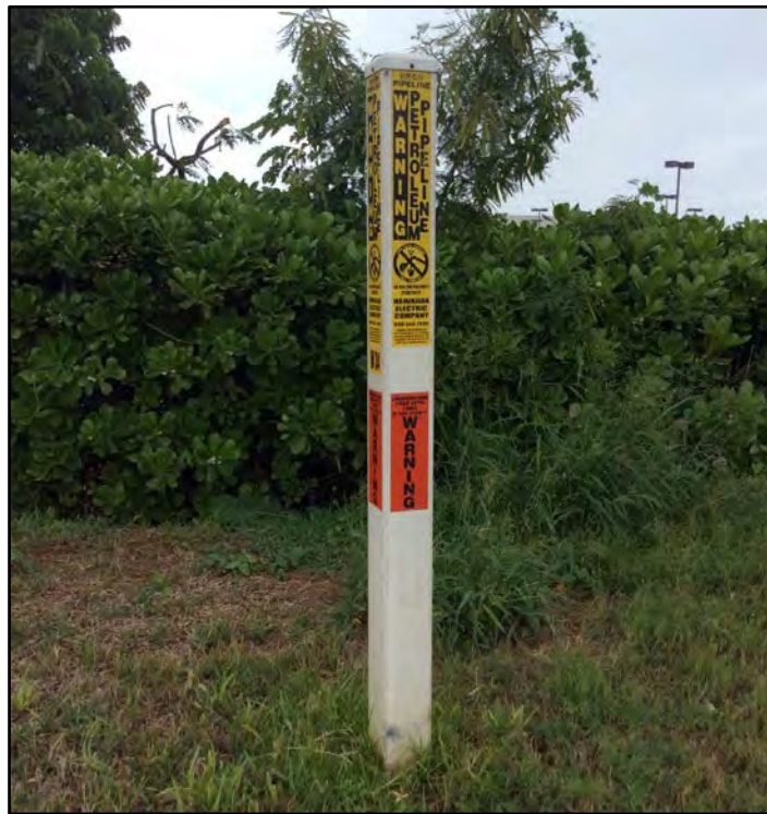
Figure 28. Petroleum pipeline warning signpost off makai /east corner of Kapolei Parkway and Kalaeloa Boulevard intersection, view to southeast
