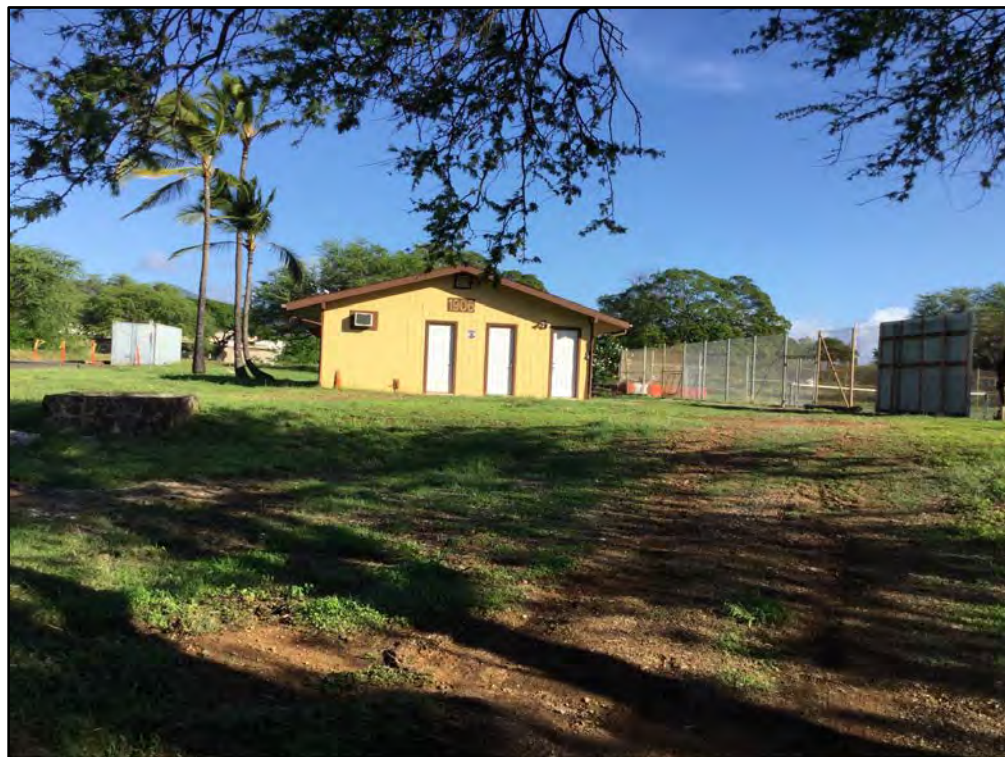
Figure 88. Building associated with tennis courts along Wākea Street segment, view to north
