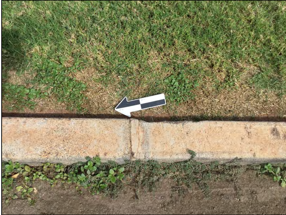
Figure 83. Potentially historic curb, along Hornet Street segment, close-up view
