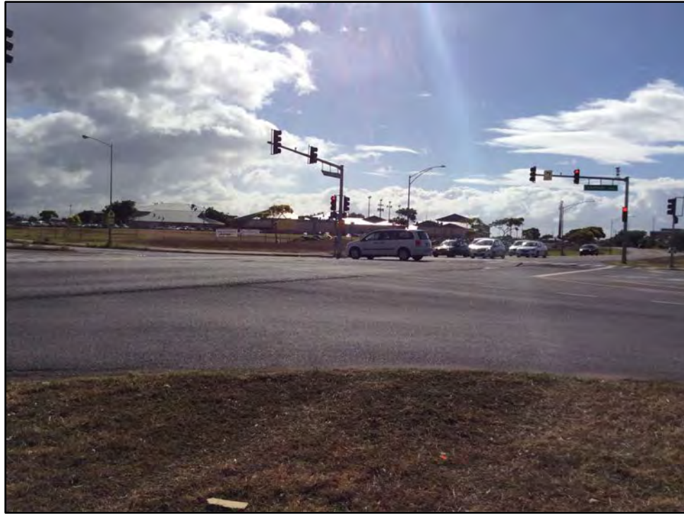
Figure 35. General view of the intersection of Fort Barrette Road and Kapolei Parkway, view to east
