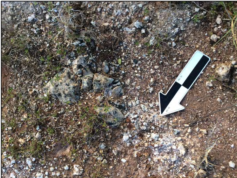
Figure 80. In situ concrete in CSH 1 Feature 18, along Copahee Avenue segment, close-up view
