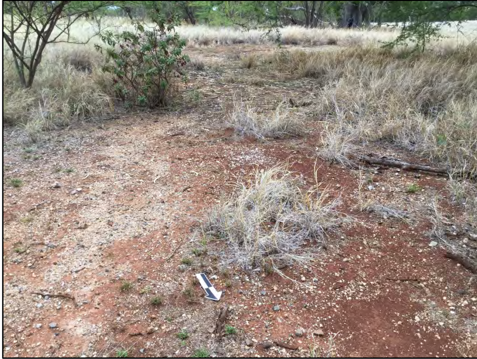
Figure 46. CSH 1 Feature 3 former foundation area, along Roosevelt Avenue segment, view to south
