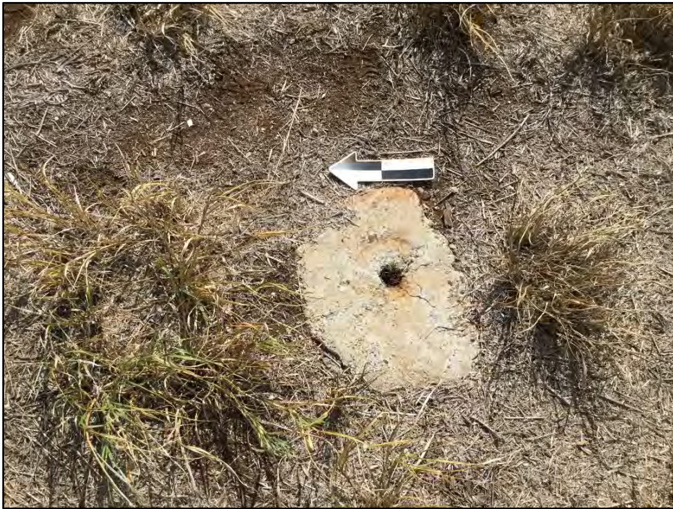
Figure 66. Concrete and metal postholes on north side of CSH 1 Feature 13, along Kamōkila Boulevard segment, view to east
