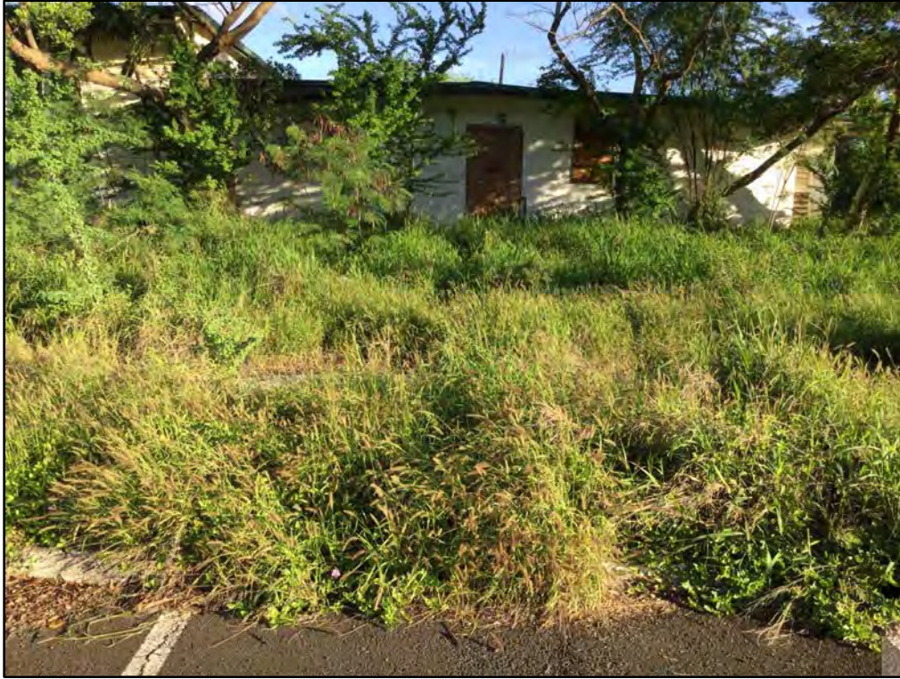
Figure 95. Abandoned buildings along Road A segment, view to north
