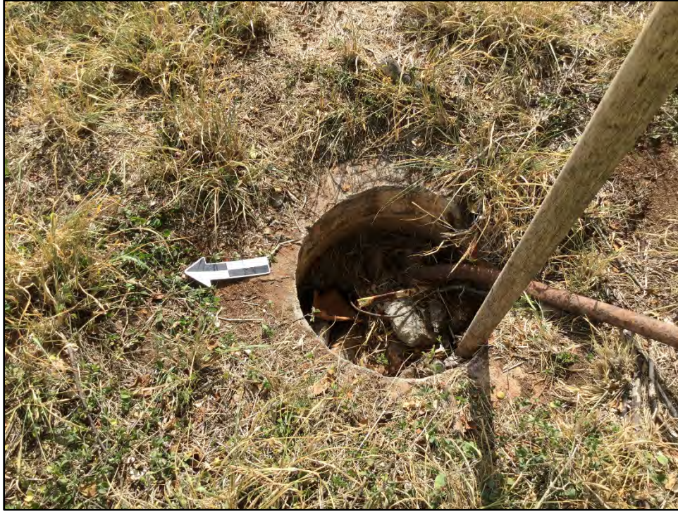
Figure 65. Concrete depression off of southwest corner of CSH 1 Feature 13, along Kamōkila Boulevard segment, view to east
