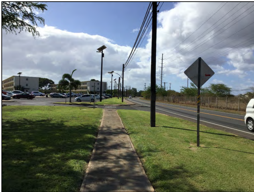
Figure 41. General view of Roosevelt Avenue from Franklin Street, view to west
