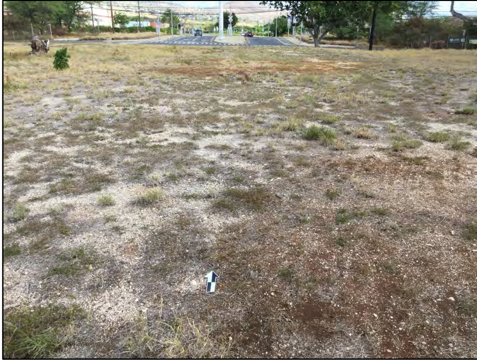
Figure 61. CSH 1 Feature 10 former foundation area, along Kamōkila Boulevard segment, view to north
