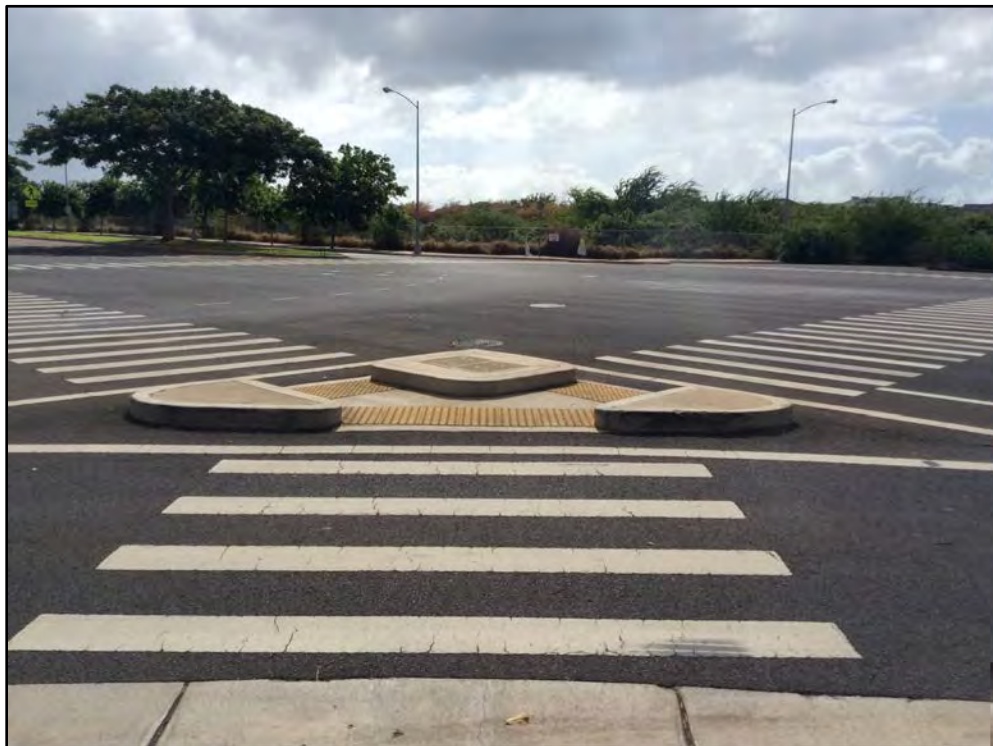
Figure 32. General view of the intersection of Kapolei Parkway and Wākea Street, view to east
