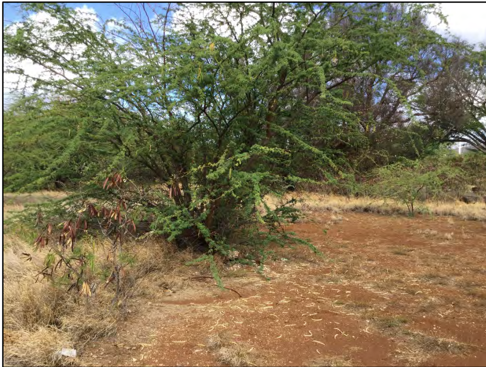
Figure 72. CSH 1 Feature 16 former foundation area, along Kamōkila Boulevard segment, view to west
