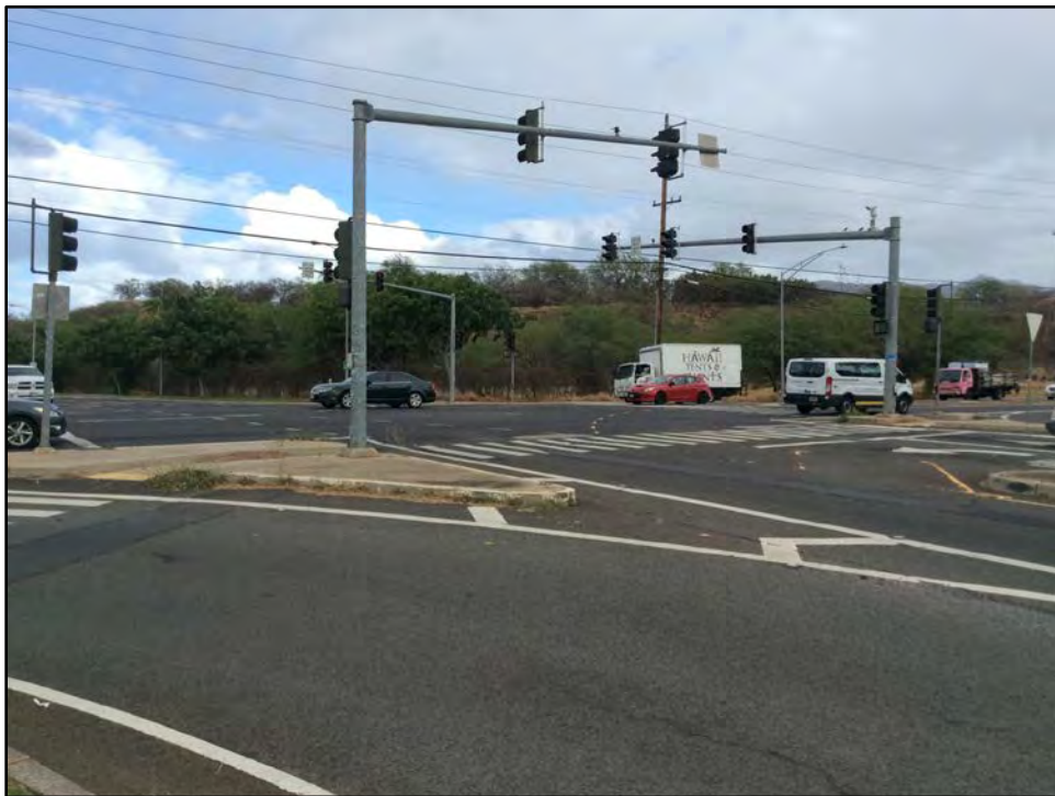
Figure 38. General view of the intersection of Fort Barrette Road and Kama'aha Avenue, view to west
