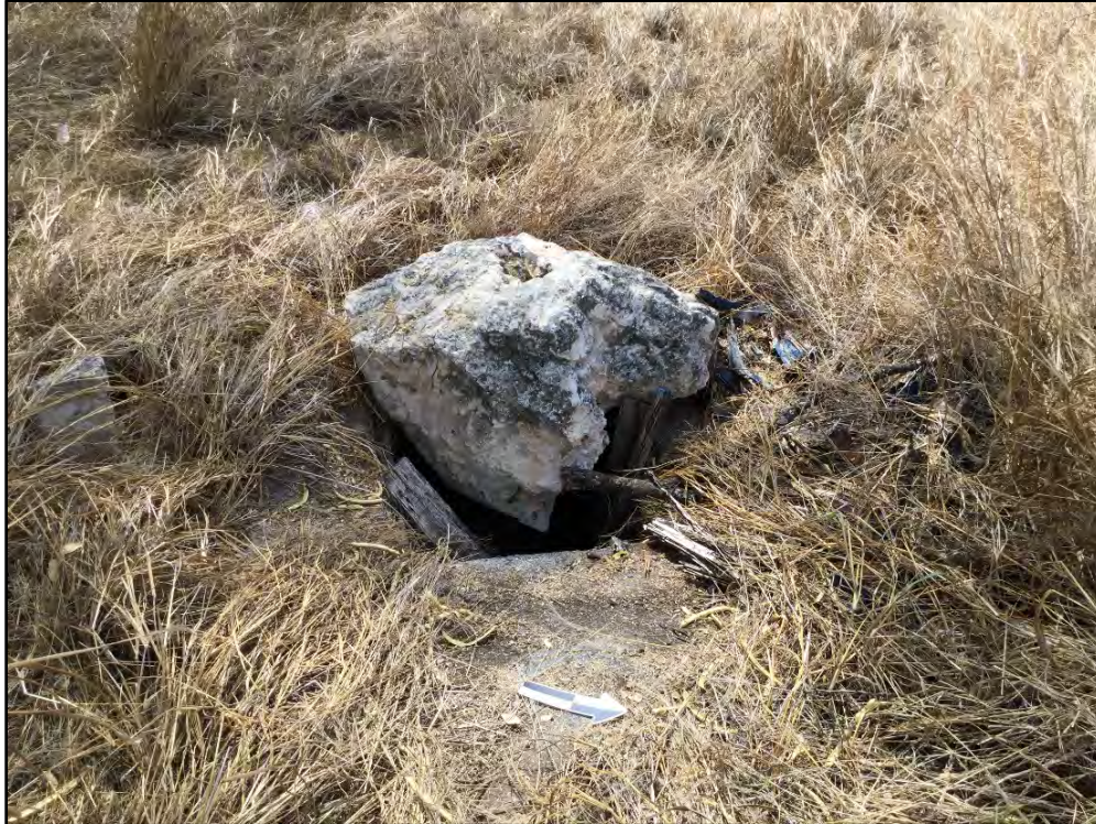
Figure 101. Concrete drainage, along Saratoga Avenue segment, view to southwest
