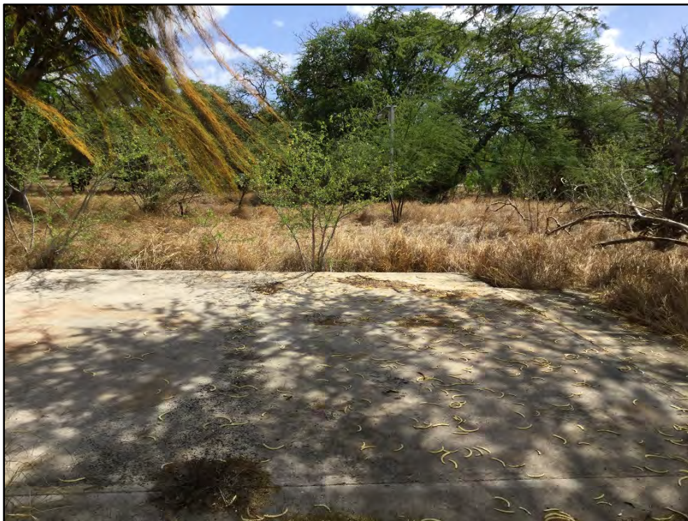
Figure 100. Modern concrete slab interconnected with sidewalks, note modern light post, along Saratoga Avenue segment, view to north
