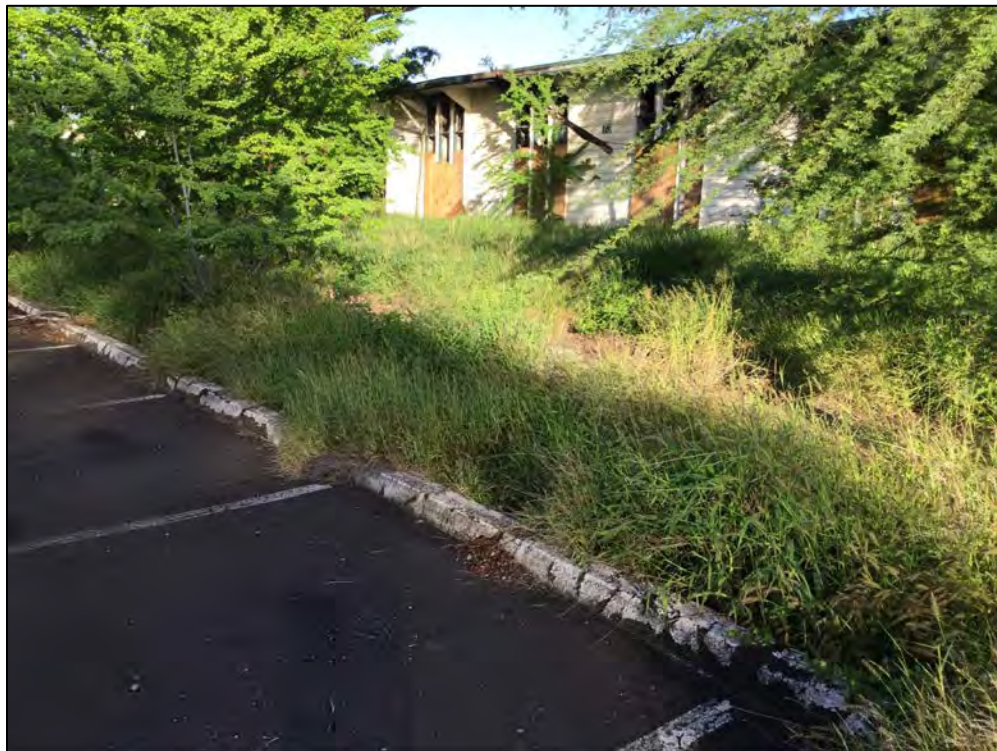
Figure 96. Abandoned buildings along Road A segment, view to northwest
