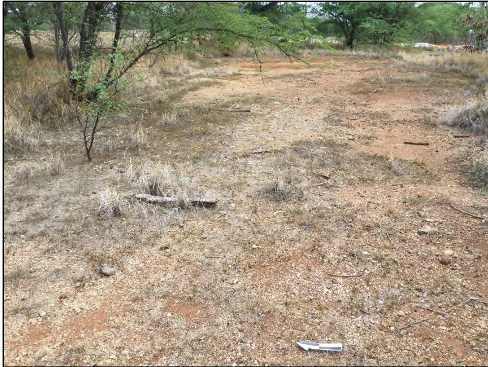
Figure 57. CSH 1 Feature 9 former foundation area, along West Perimeter Road segment, view to east
