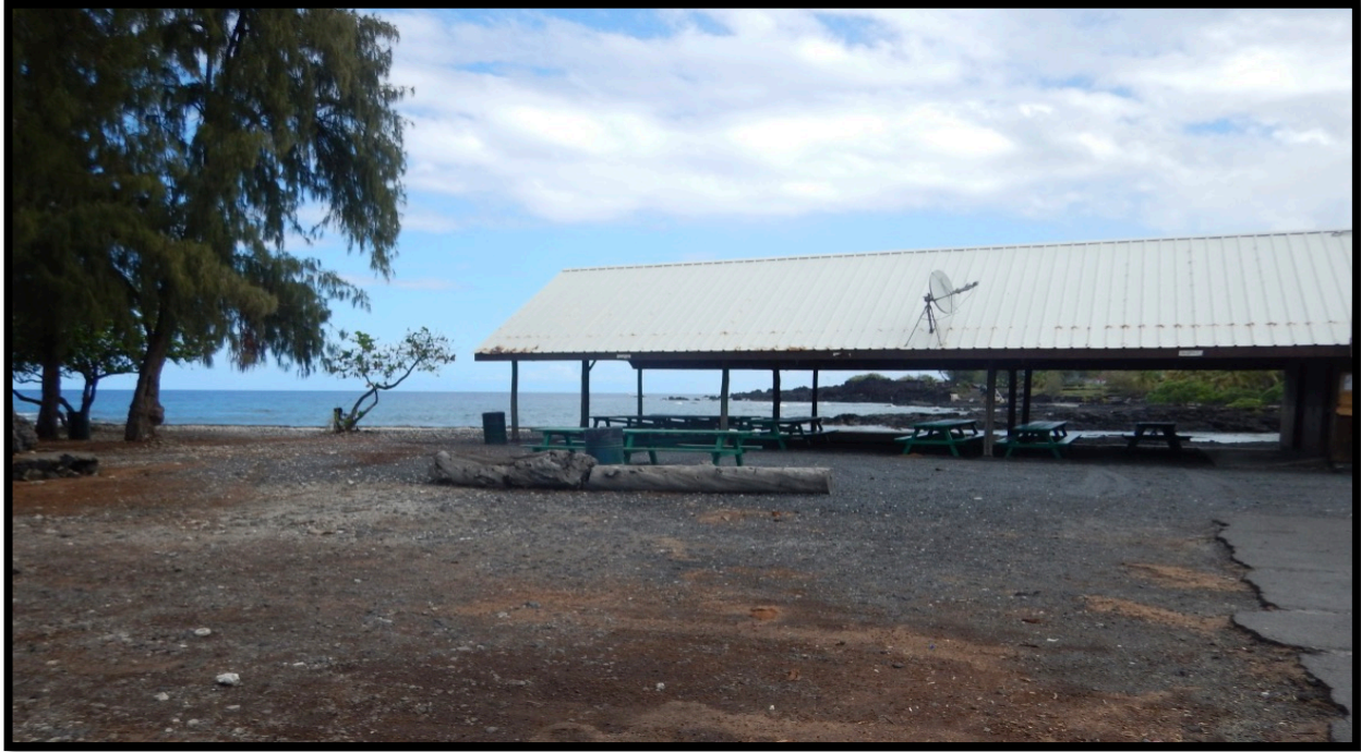
Exhibit 2.1 – View of the existing pavilion and edge of parking area from the basketball court.
