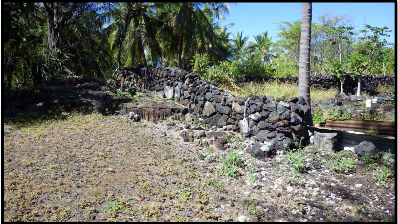
Figure 30. Site 31098, Segment 2 wall (view to southwest)
