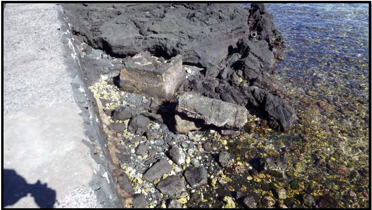
Figure 29. Concrete pier block (view to west)
