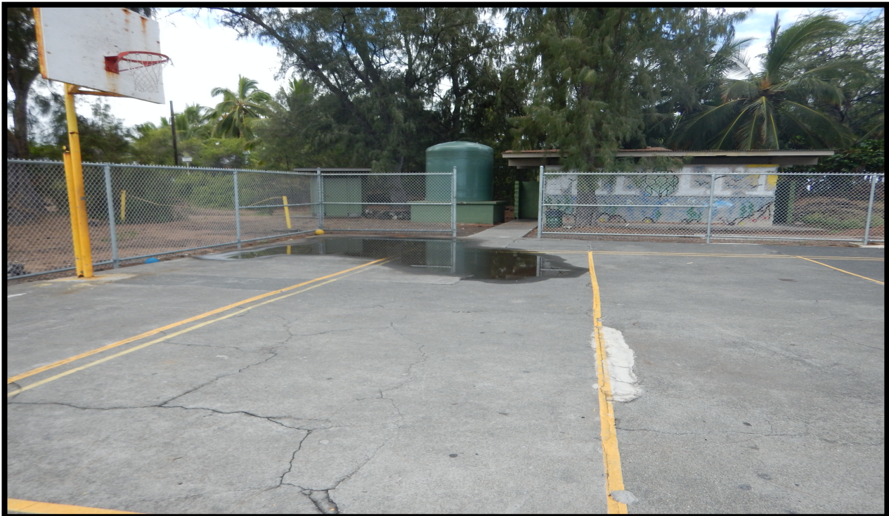
Exhibit 2.3 – View of the basketball court and comfort station in the background.
