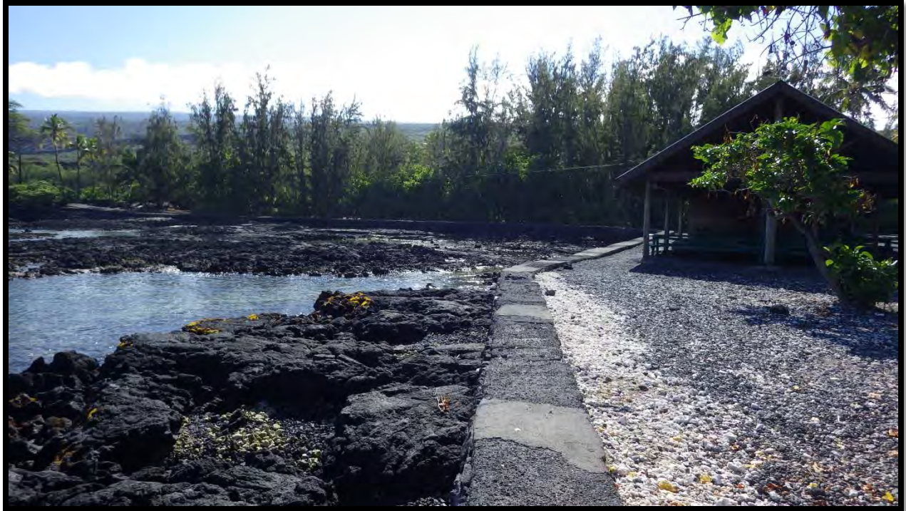
Figure 28. Site 31097 retaining wall (view to northeast)
