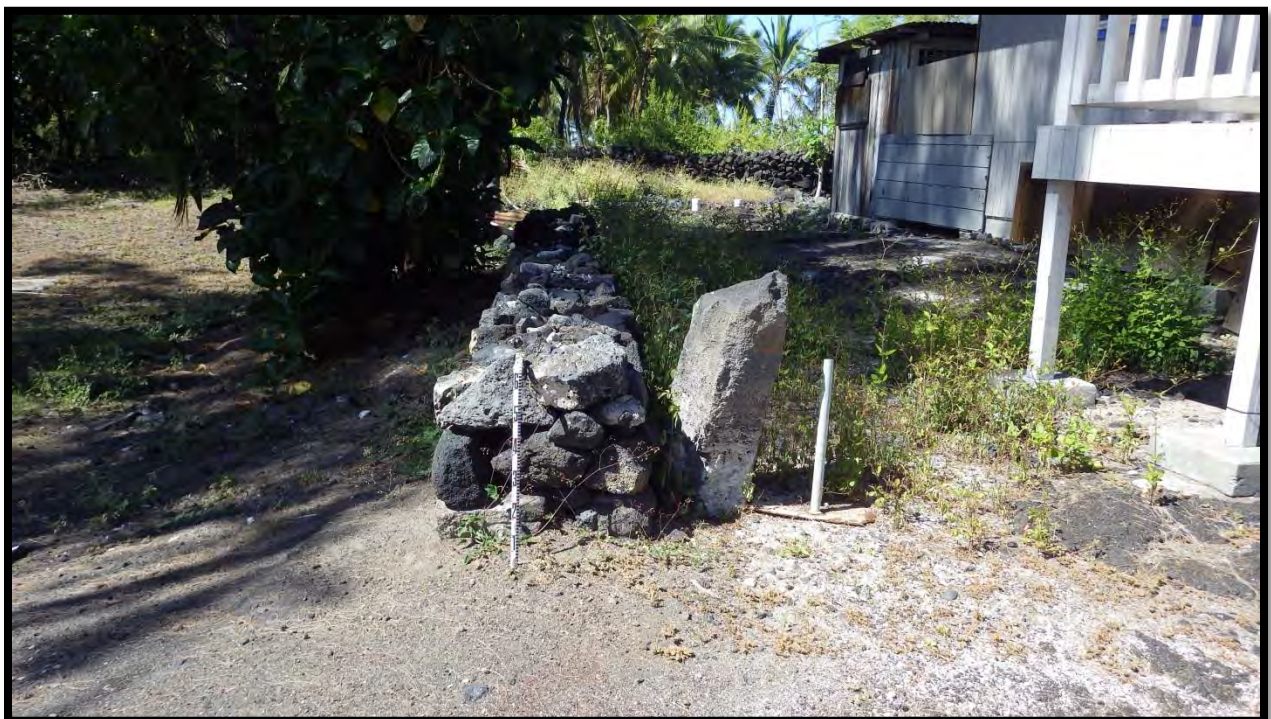
Figure 31. Site 31098, Segment 3 wall (view to south)
