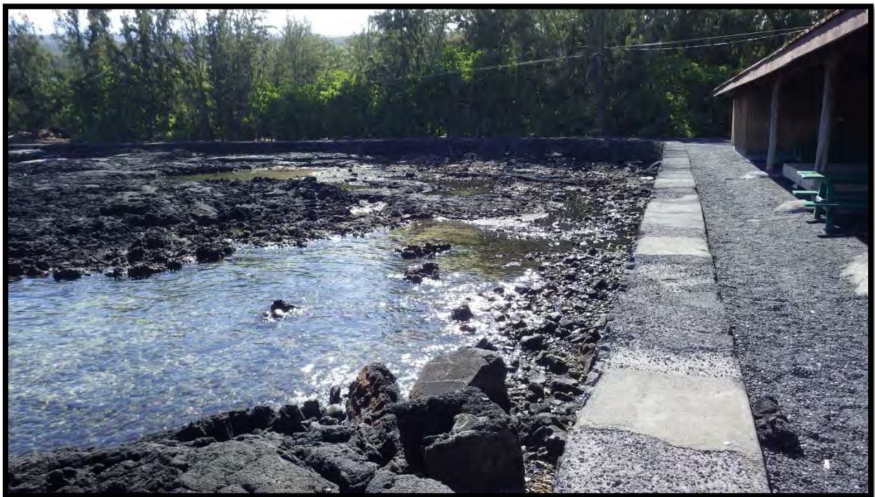
Figure 27. Site 31097 retaining wall (view to east)
