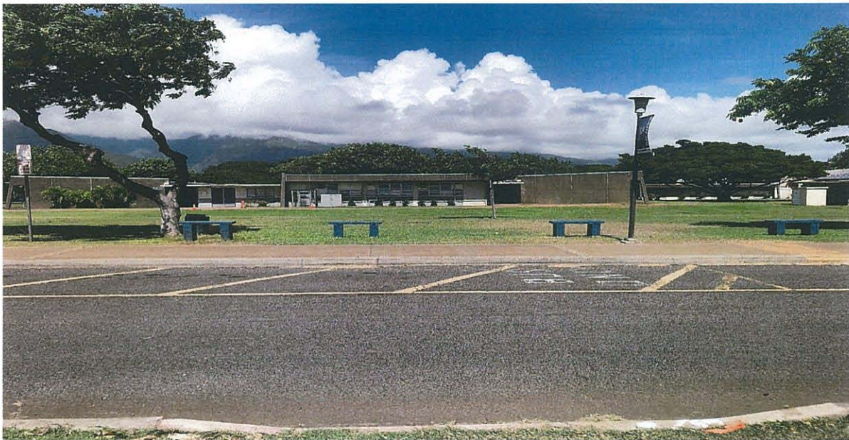
Photograph 1. West View of Building Site from Driveway. Building A in Background.
