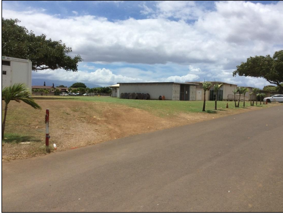
Figure 30. Overview of portable classrooms near the Staff Parking Lot, south of the Student Parking Lot, view to southeast
