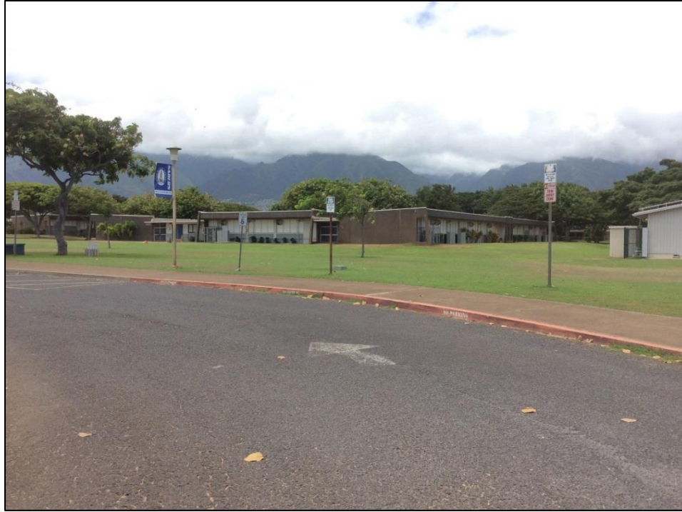
Figure 48. Overview of Maui High School campus fronting Lono Avenue, view to west
