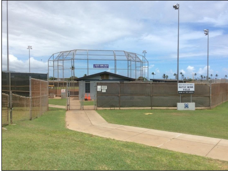
Figure 32. Entrance to the Patsy Mink Field baseball field on the western side of the Student Parking Lot, view to northwest
