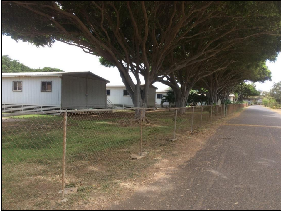
Figure 42. Overview of portable classrooms along the western side of the school campus, view to south
