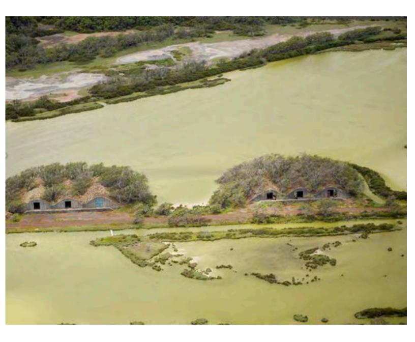
This picture shows camouflaged elevated Quonsets installed as a munitions store in Kahahā pond. A grid circuit of stone and macadam access revetments are just wide enough for military transport vehicles.
