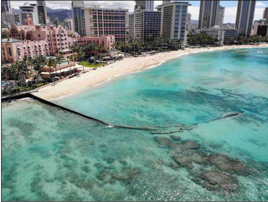
Figure 1-6 Conditions before replacement of Royal Hawaiian groin
