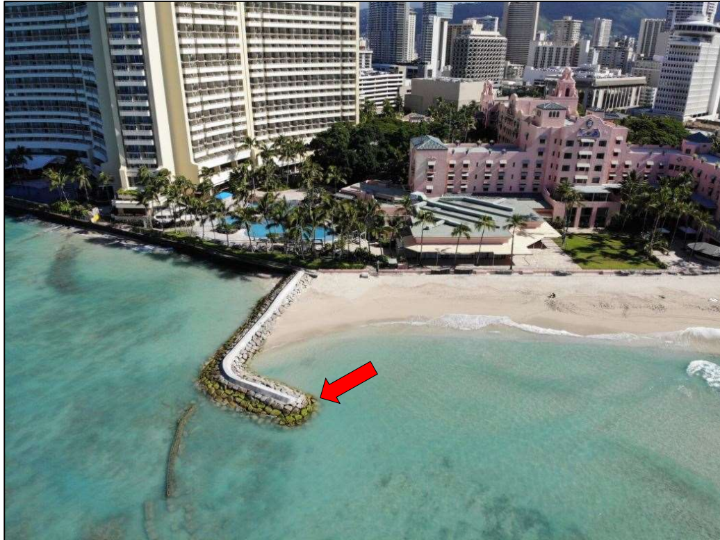
Figure 1-7 Conditions after replacement of Royal Hawaiian groin (Aug 2020)
