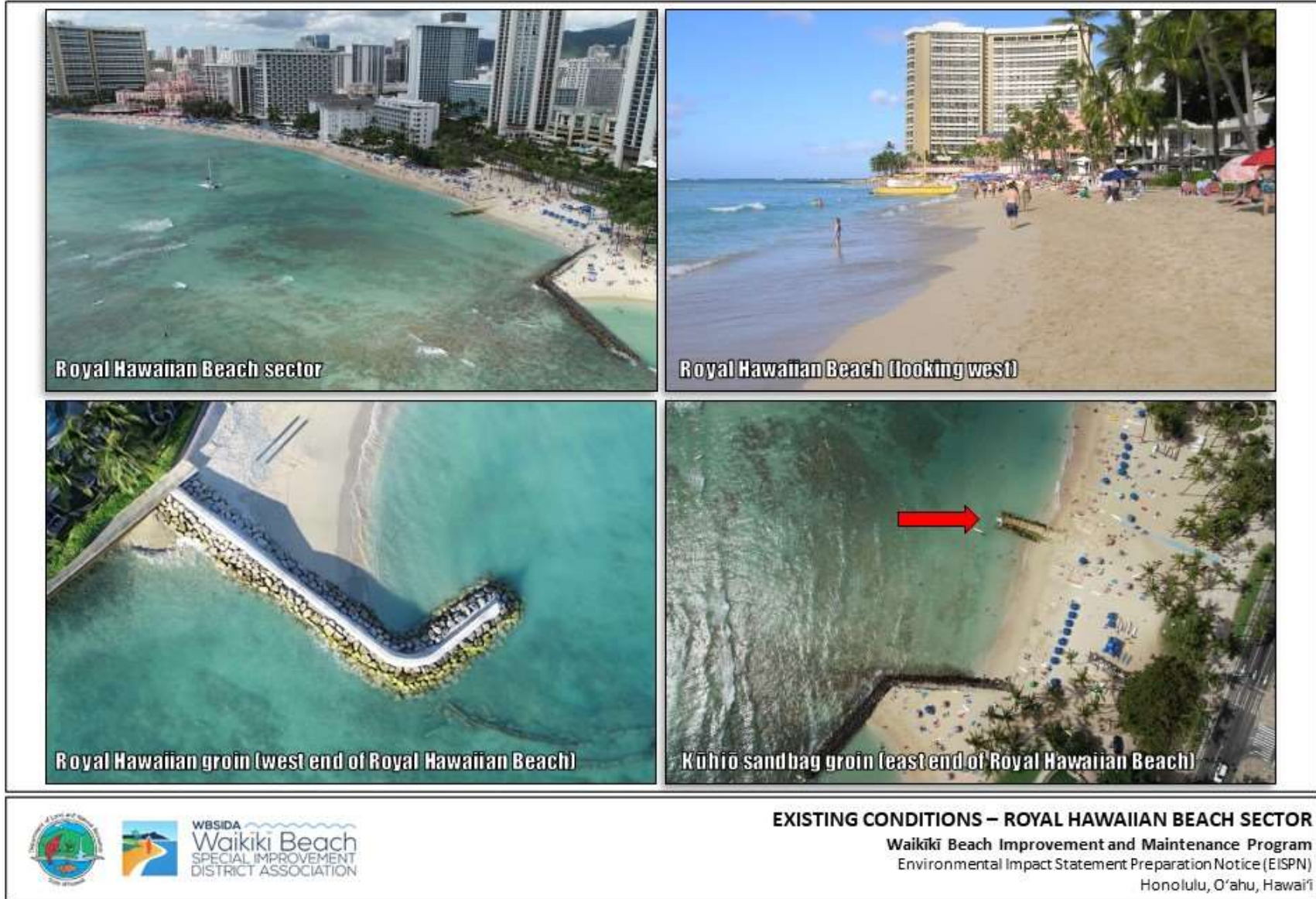
Figure 5-5 Existing conditions – Royal Hawaiian Beach sector
