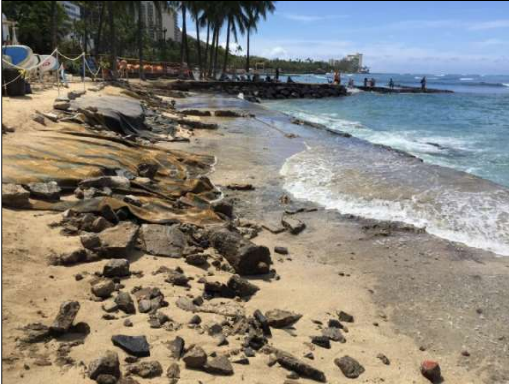
Figure 1-4 Conditions before construction of Kūhiō Sandbag Groin
