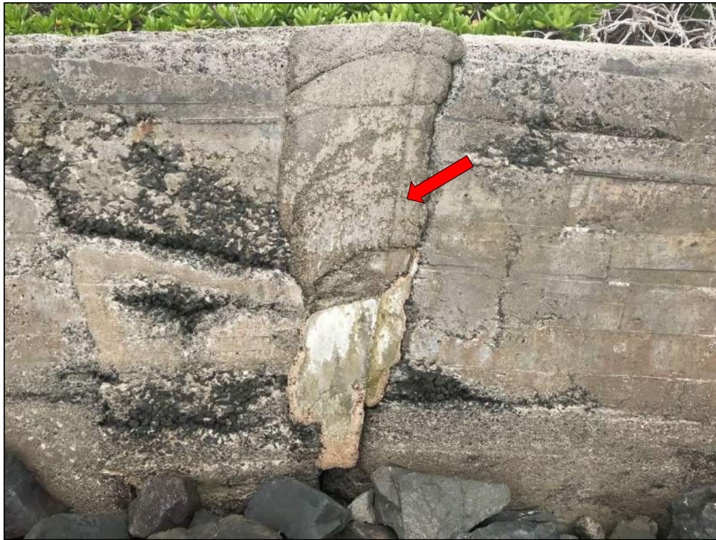
Figure 2-6 Concrete repairs at panel joint (July 2020)
