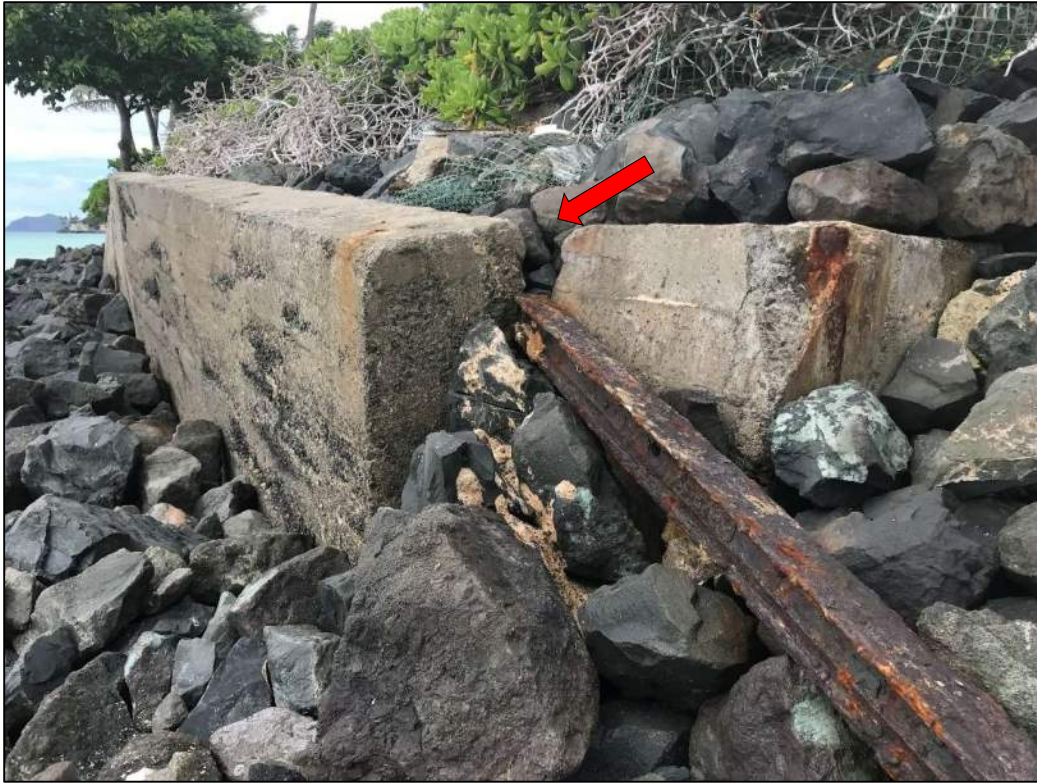
Figure 2-10 Disconnected return at north end of seawall (July 2020)
