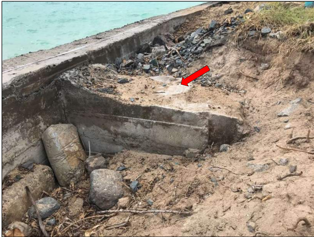
Figure 2-4 Counterfort on inshore side of seawall (July 2020)
