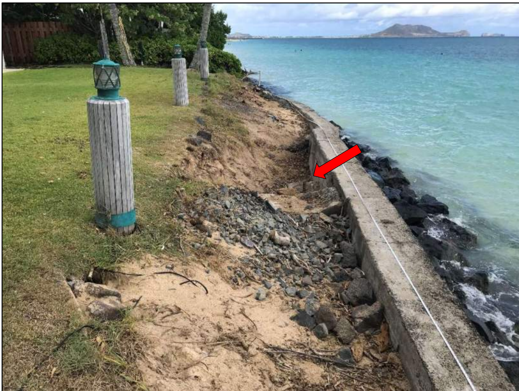
Figure 2-11 Sinkholes inshore of existing seawall (July 2020)
