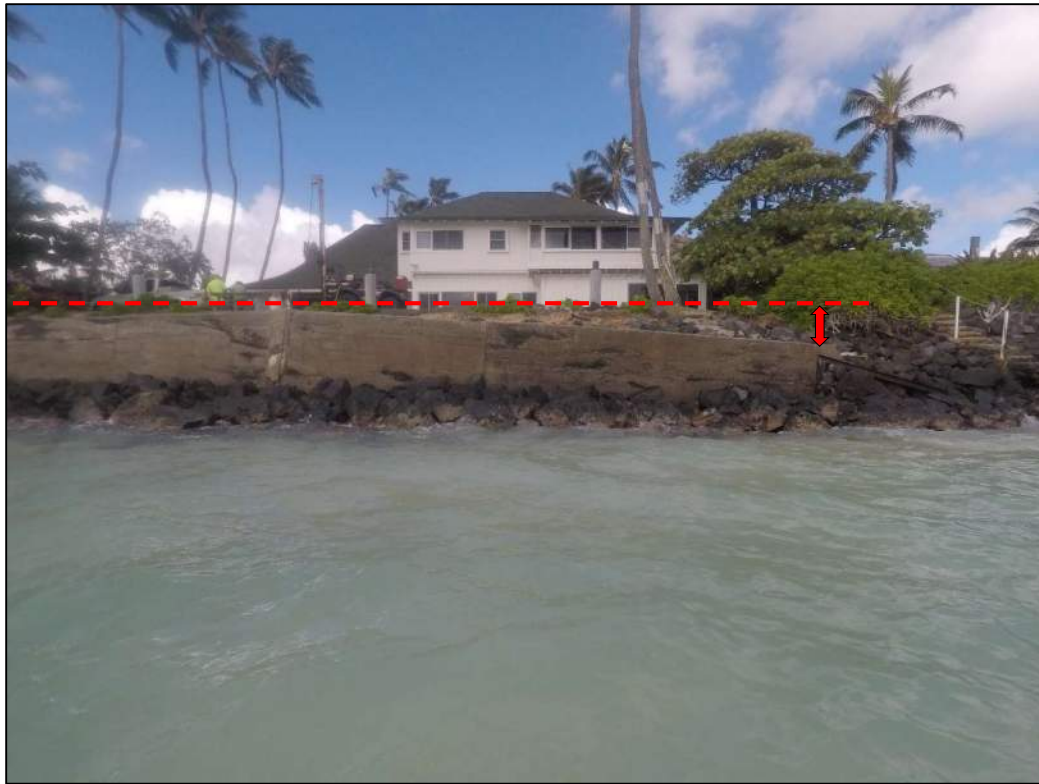
Figure 2-8 Settlement along northern portion of seawall (July 2020)
