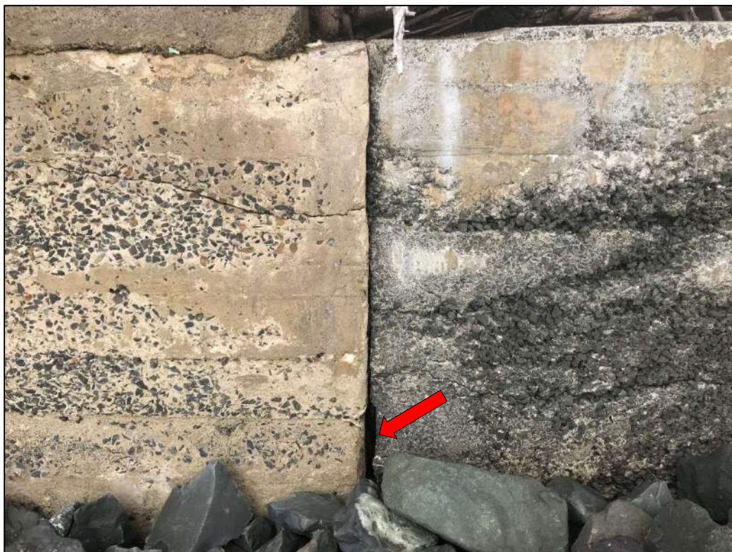
Figure 2-7 Gap between subject seawall and south adjacent seawall (July 2020)
