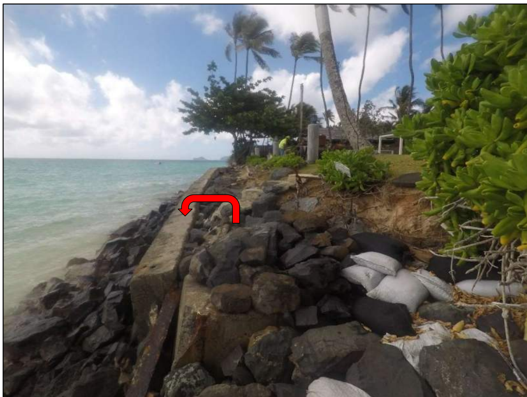
Figure 2-9 Outward rotation along northern portion of seawall (July 2020)
