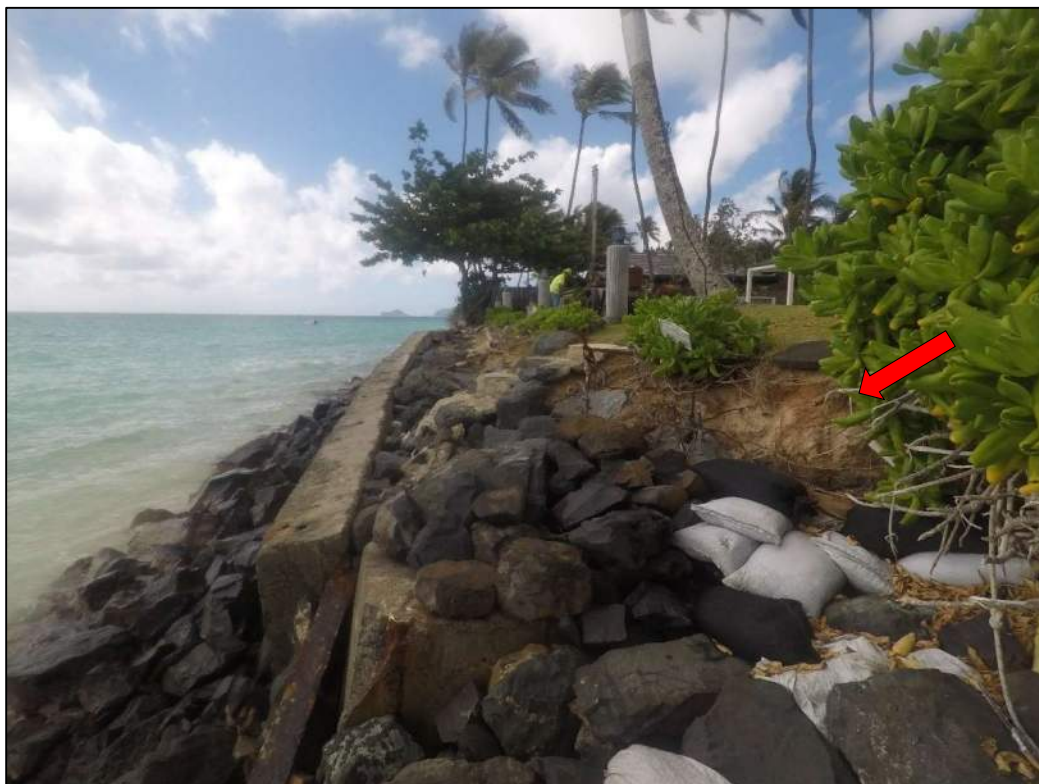
Figure 2-5 Backshore erosion along north end of shoreline (July 2020)
