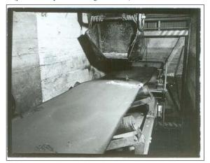
Figure 60. Photo of interior water damage to the bulk sugar conveyor system at Kahului Harbor caused by the 1960 tidal wave (photo courtesy of HC&S Sugar Museum)
