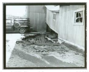
Figure 38. Photograph (1960) of damage to bulk sugar conveyor system at Kahului Harbor following a tidal wave; note extensive ground utilities under pavement surface to support the harbor infrastructure (photo courtesy of HC&S Sugar Museum)
