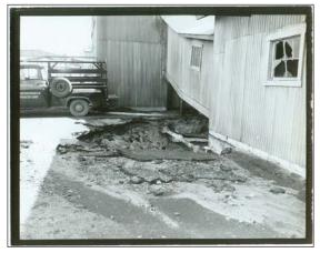
Figure 58. Photograph (1960) of damage to bulk sugar conveyor system at Kahului Harbor following a tidal wave; note extensive ground utilities under pavement surface to support the harbor infrastructure (photo courtesy of HC&S Sugar Museum)
