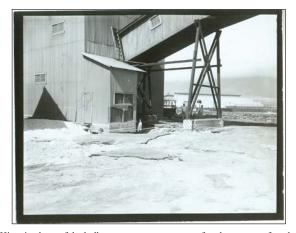
Figure 37. Historic photo of the bulk sugar conveyor system after the concrete foundation was undermined by a 1960 tidal wave (photo courtesy of HC&S Sugar Museum)
