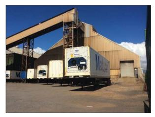
Figure 77. General view of the east end of CSH 1 showing steel framing supporting a bulk sugar conveyor system (CSH 4), view to west
