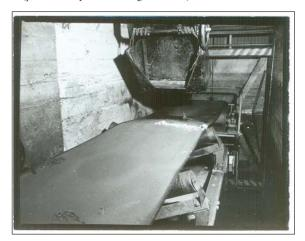
Figure 40. Photo of interior water damage to the bulk sugar conveyor system at Kahului Harbor caused by the 1960 tidal wave (photo courtesy of HC&S Sugar Museum)
