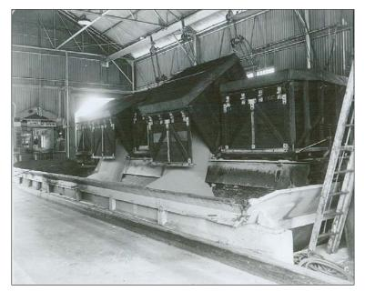
Figure 86. Circa 1950s photograph of the interior CSH 2 while still in operation; note framing; unrefined sugar is being transported into the storehouse via the conveyor system (courtesy of HC&S Sugar Museum)
