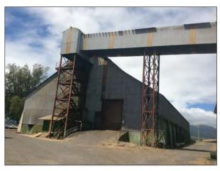
Figure 93. General view of the southwest side of CSH 3 showing architectural features, including concrete columns supporting steel structure and conveyor, view to southwest
