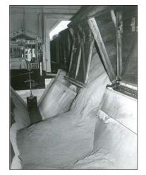
Figure 34. Interior of storehouse (CSH 2) while in operation circa 1950s, showing bulk unrefined sugar being transported to the storehouse from the intake conveyor system (photo courtesy of HC&S Sugar Museum)
