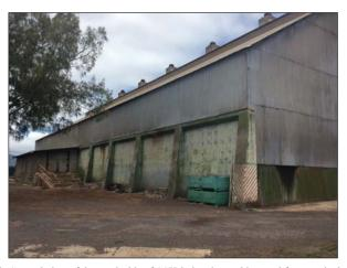
Figure 92. General view of the south side of CSH 3 showing architectural features, including concrete columns supporting steel structure, view to north
