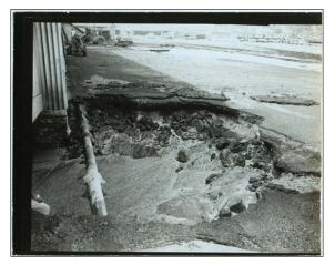
Figure 39. Photo of utilities exposed at Kahului Harbor Bulk Sugar plant following a 1960 tidal wave (photo courtesy of HC&S Sugar Museum)
