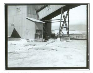
Figure 57. Historic photo of the bulk sugar conveyor system after the concrete foundation was undermined by a 1960 tidal wave (photo courtesy of HC&S Sugar Museum)
