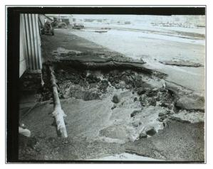
Figure 59. Photo of utilities exposed at Kahului Harbor Bulk Sugar plant following a 1960 tidal wave (photo courtesy of HC&S Sugar Museum)
