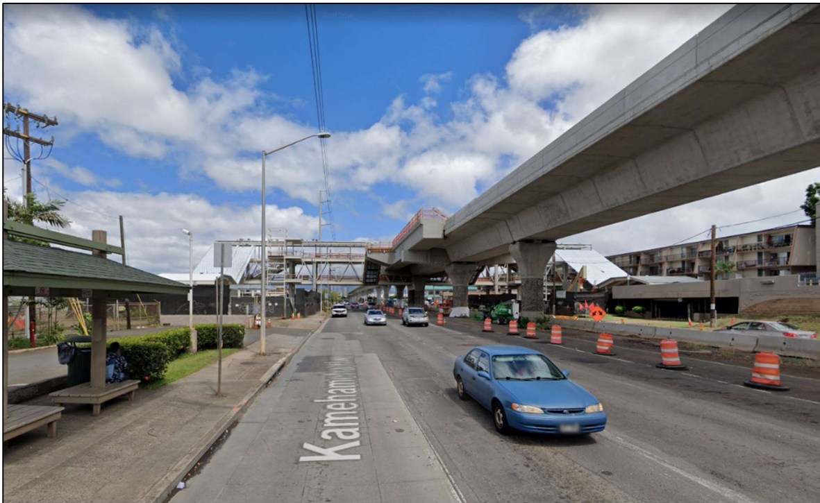
Figure 3.9 View of Makai side of Kamehameha Highway and Kaonohi Street (Looking West)
