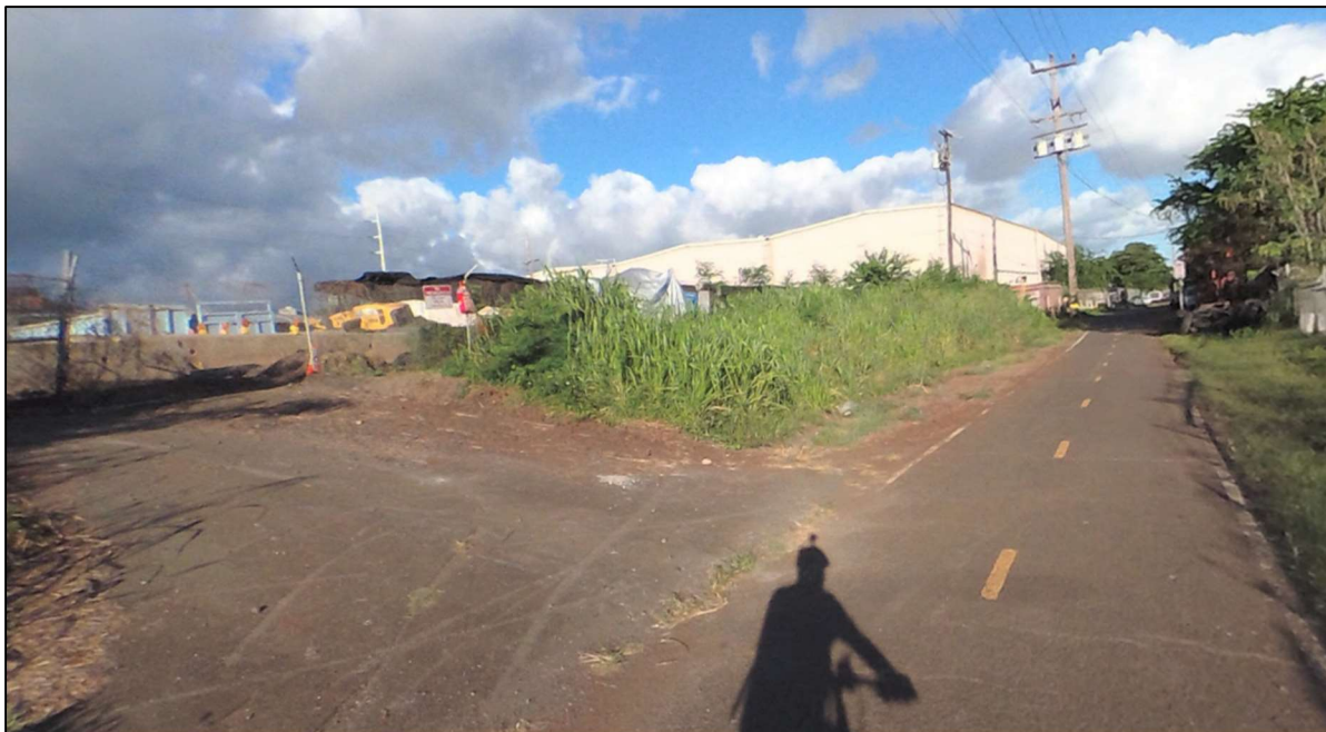
Figure 3.11 View of Pearl Harbor Bike Path (Project Site at the left)
