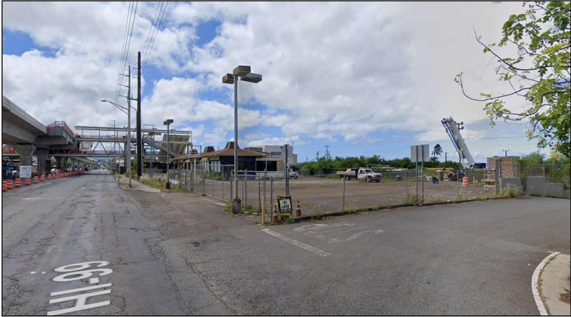
Figure 3.6 View of Kamehameha Highway at Project Site (Looking East)
