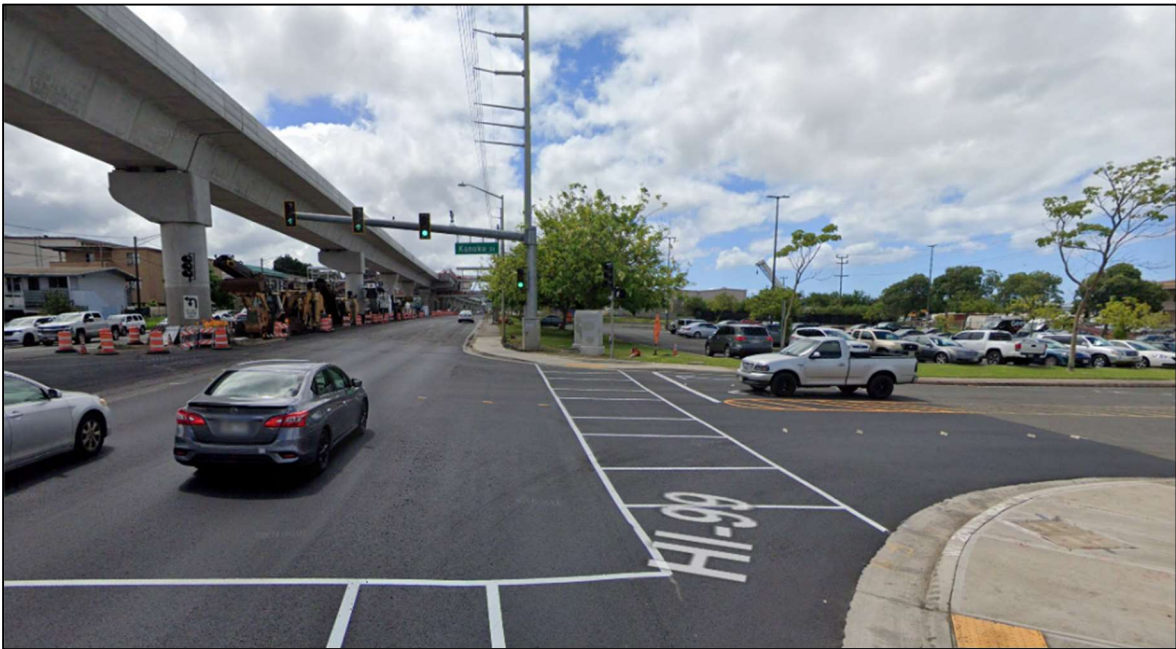
Figure 3.10 View of Kamehameha Highway at Kanuku Street (Looking East)
