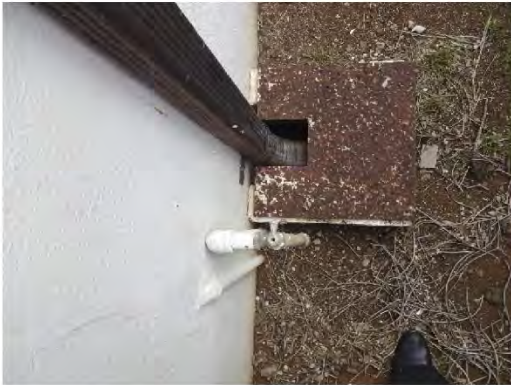
Photo 3 Downspout to underground
