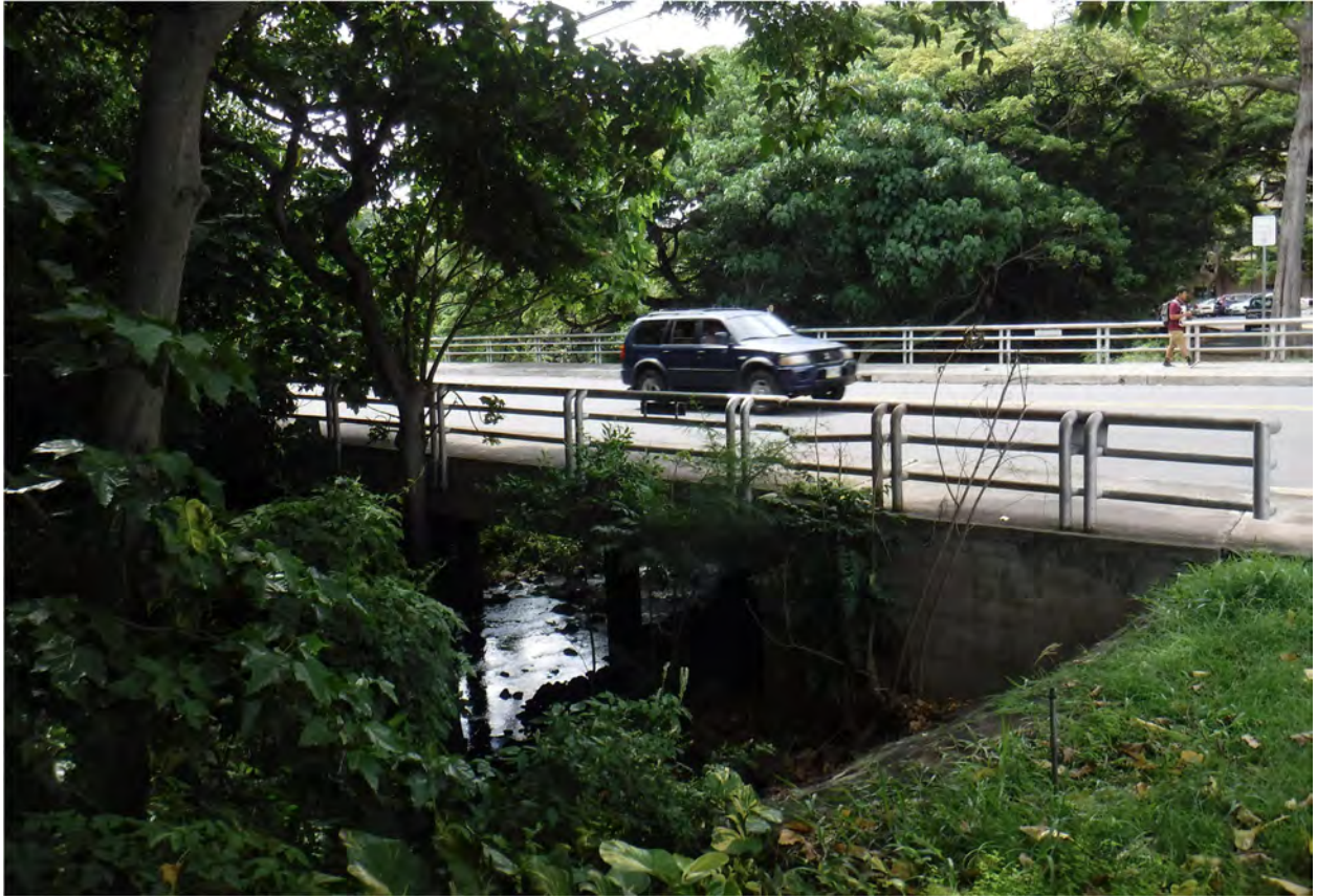
Dole Street Bridge at Mānoa Stream
