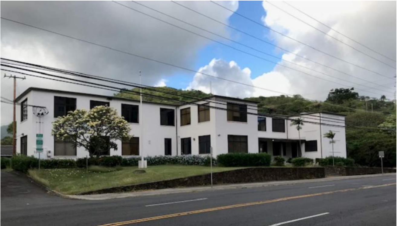
View of the former Laboratory and Administration Building fronting Dole. (Source: MASON)
