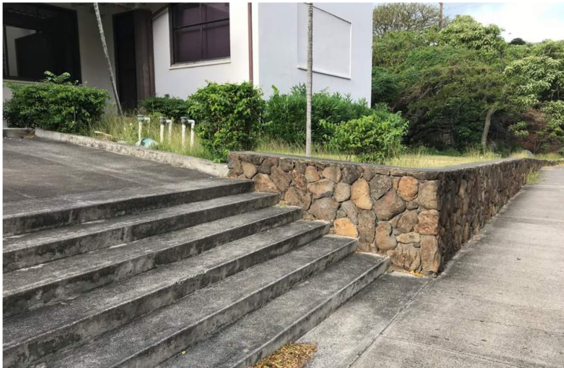
Original stair and rock wall at front entrance. (Source: MASON)
