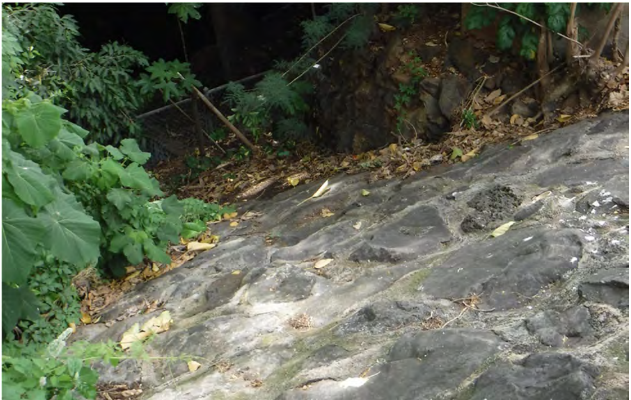
Mānoa Stream, Rip-Rap Embankment
