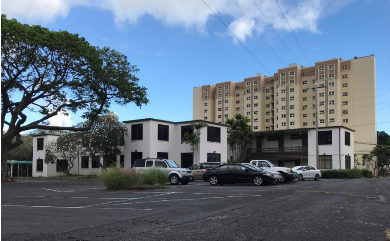
Rear view of former Laboratory and Administration Building. (Source: MASON)
