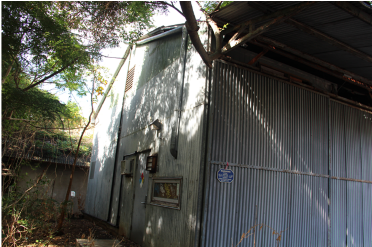
Annex II, east end showing flush entry door and aluminum frame window.
