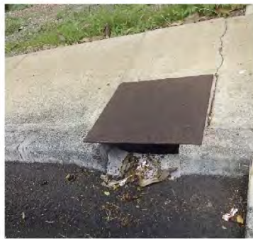
Photo 8 Curb inlet in parking lot
