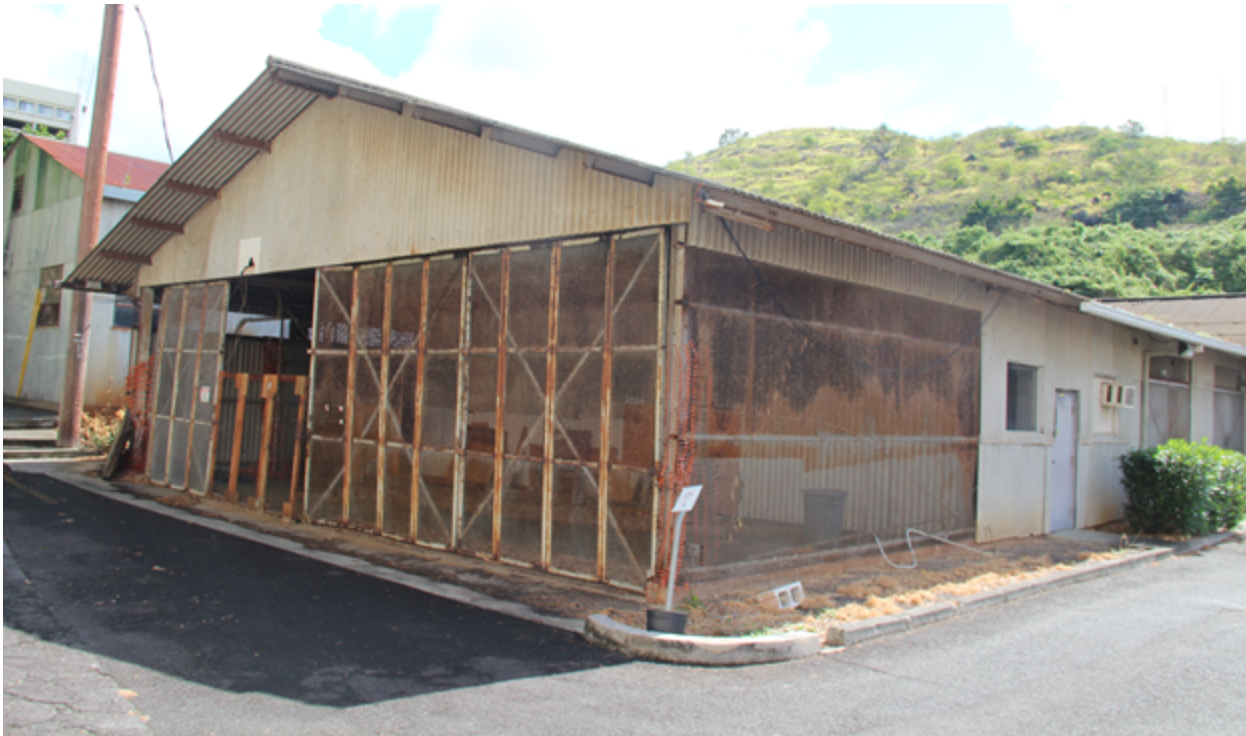
Annex I, west end showing screened area with sliding screen doors.
