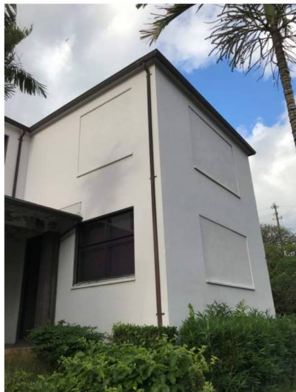
In-filled windows at front. (Source: MASON)
