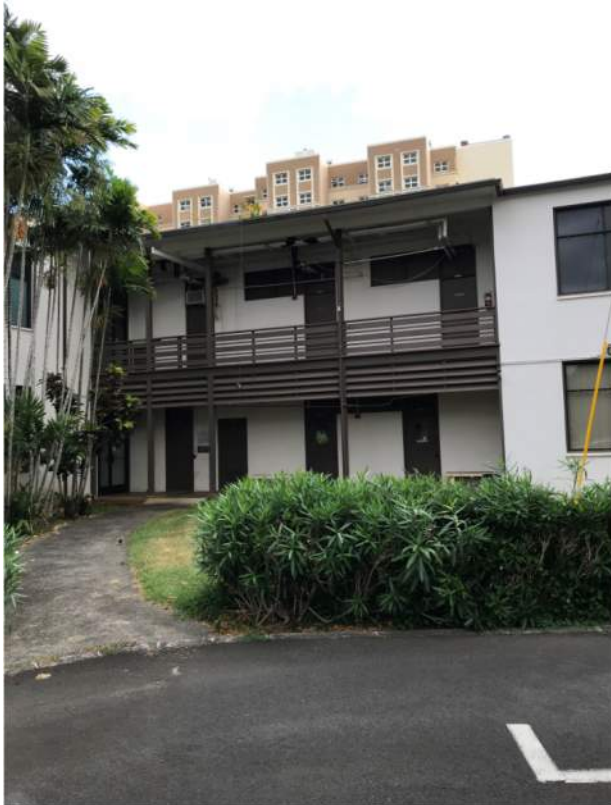
Rear walkway (Source: MASON)
