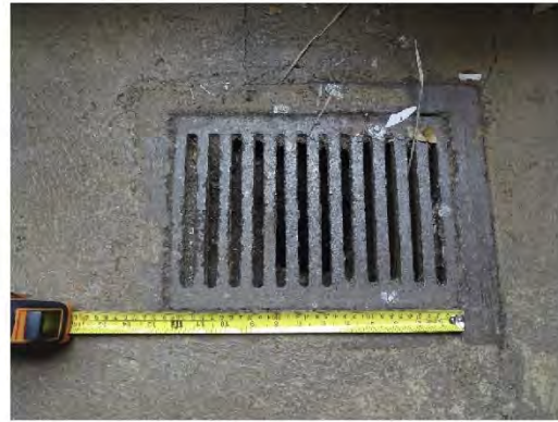
Photo 7 Inlet in east walkway
