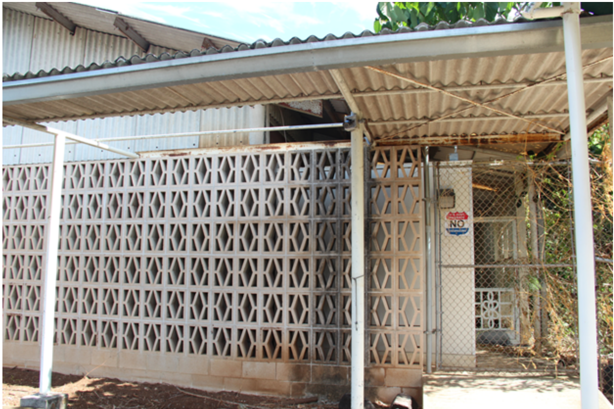
Annex I, entry to east side screened lanai showing breezeblock and chain link gate.
