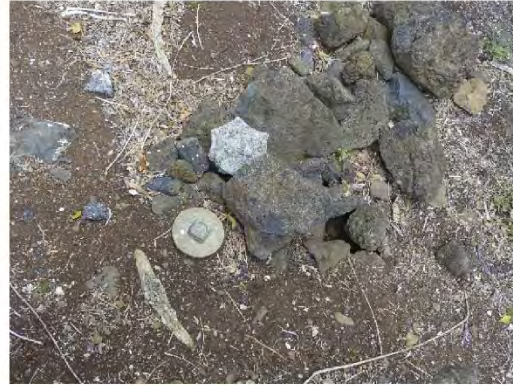
Photo 24 Sewer Cleanout at Northwest Bldg. Corner
