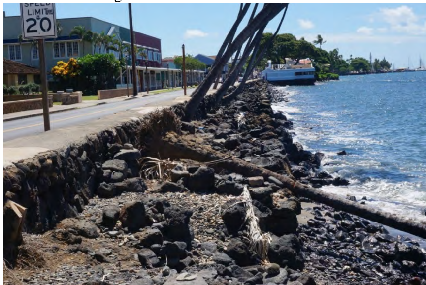
Area 2 seawall looking south
