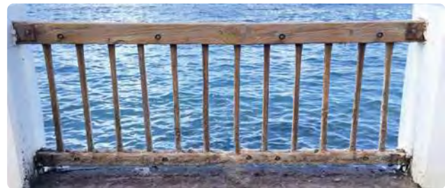
DETERIORATED RAILING
