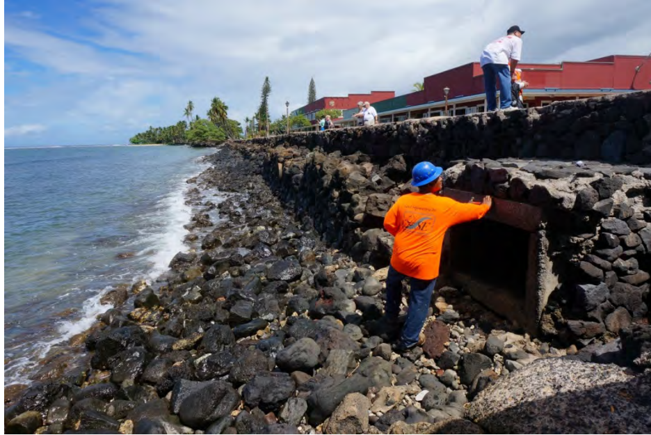
Area 2 seawall looking north.
