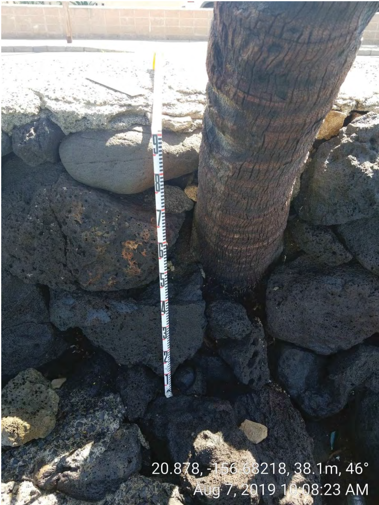
Figure 11: Photographic View of Coconut Palm Tree Growing Out of Wall Adjacent to Sidewalk in Area 2. View to Northeast.
