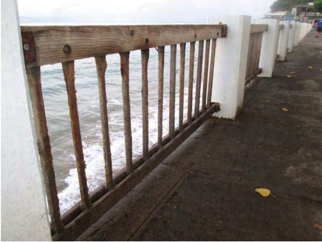
Figure 7: Existing railing on Front Street
