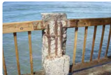
DETERIORATED POST
