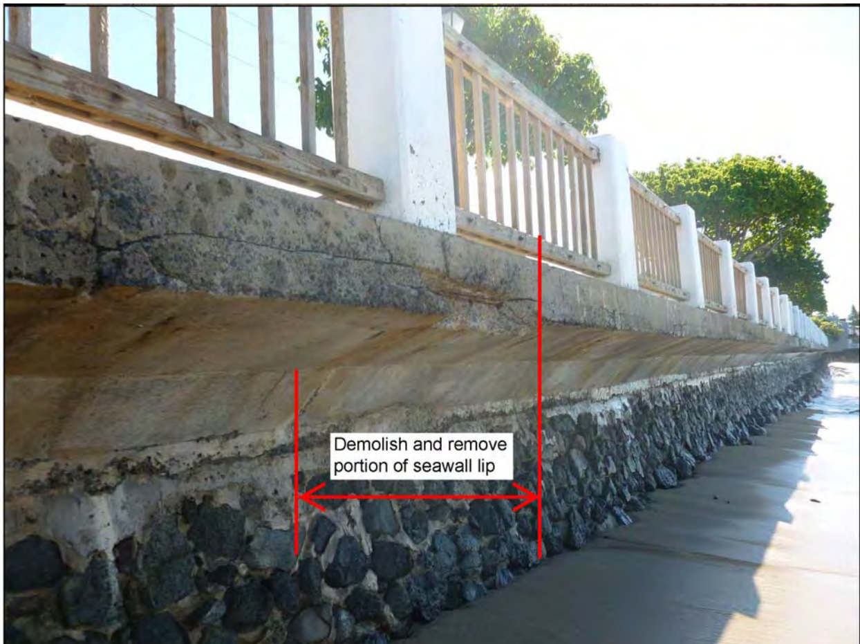
Demolish portion of overhanging lip above CRM seawall
