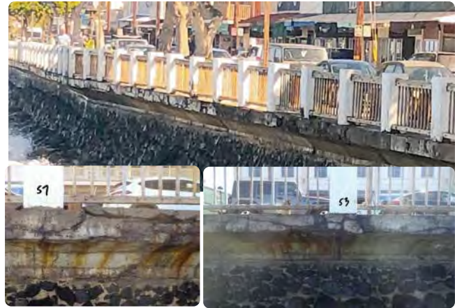
WAVE DEFLECTOR SPALLS
