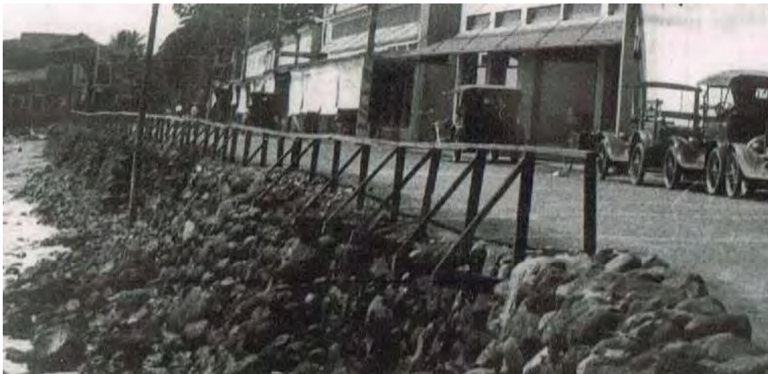
Figure 3: Railing showing detail of brace. (Maui Historical Society Collection)
