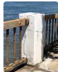
DETERIORATED RAILING
